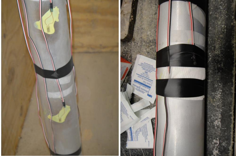
Figure 3.9 Installations and Protection of the Strain Gages
