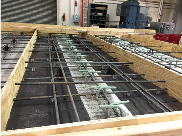
764 Fig. 4. Girder #2 prior to first concrete placement
