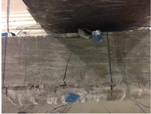
(b) Girder #1 near peak load
