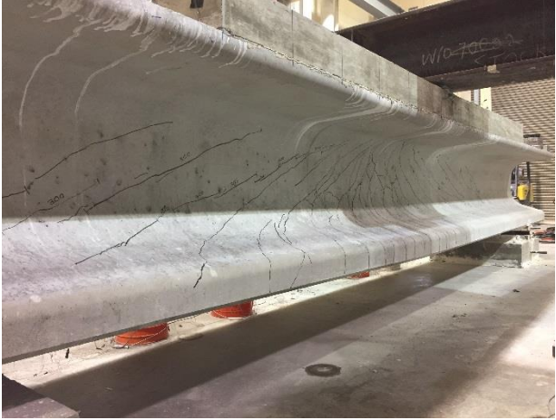
(a) Cracking at 1780 kN [400 kips] (Girder #2)
