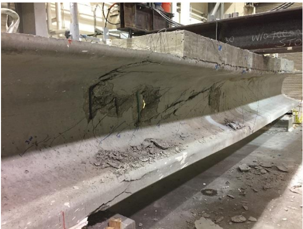
(c) Girder #1 after failure
