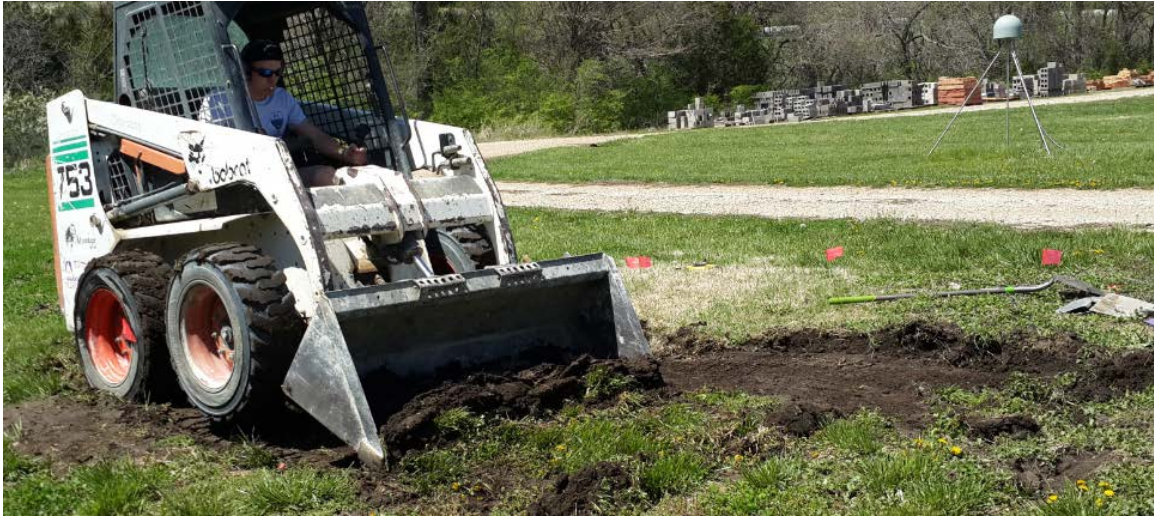
Figure 3-6 Removal of Top Soil for Extracting Subgrade Soil as Fouling Agent
