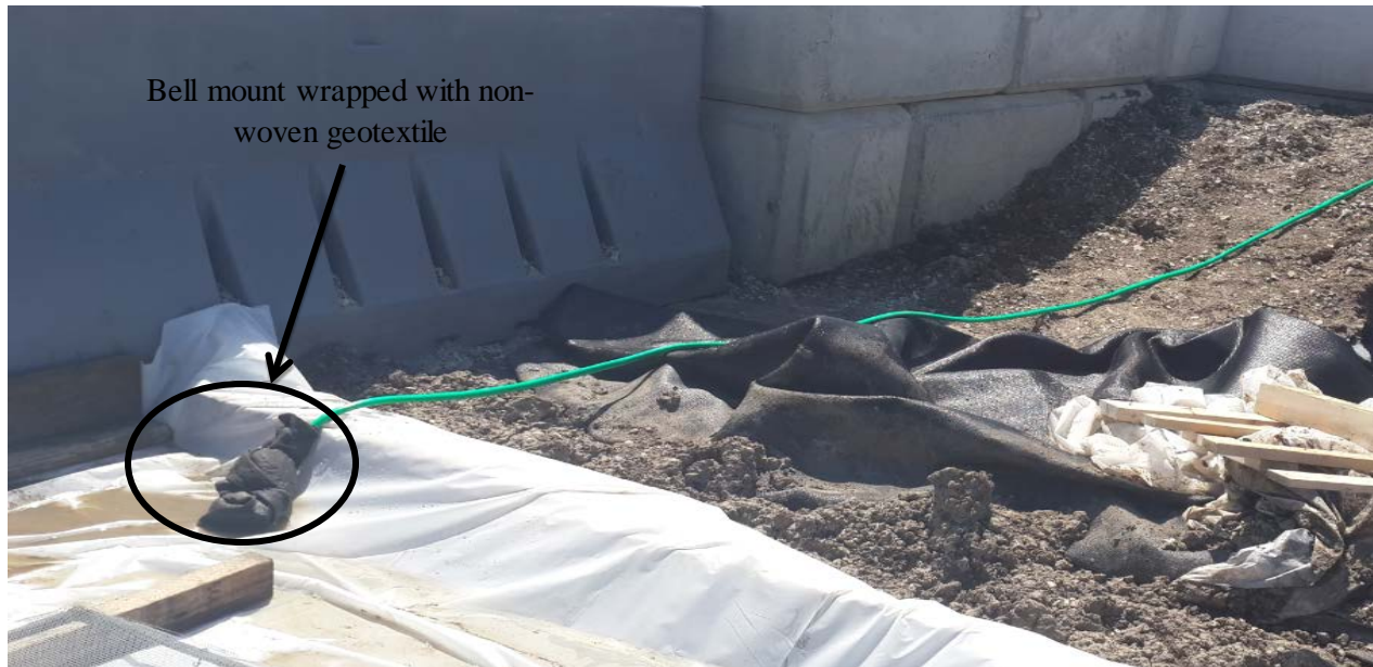
Figure 3-12 Water Drain out Arrangement after Washing Gardner Track Ballast Dust
