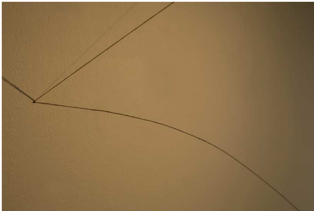
Line from Here entering gallery through wall
