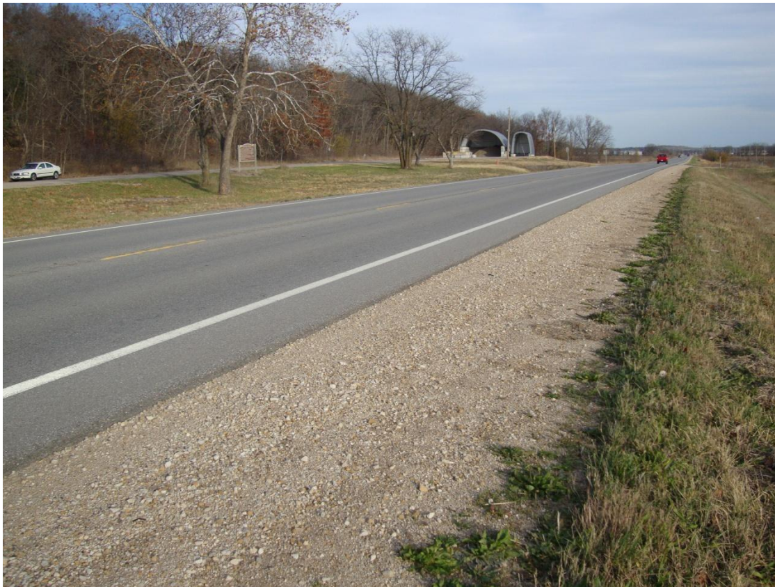
FIGURE 3 Composite shoulders on US Highway 24, Williamstown, Kansas.
