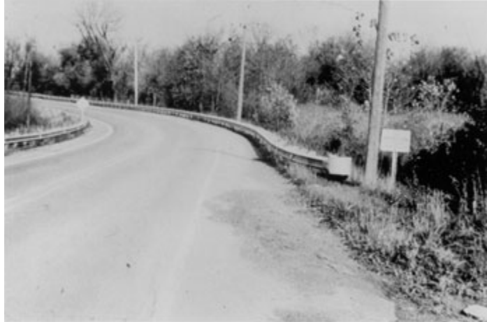
Figure 11. Typical Roadway with Roadside Hazard Rating Equal to 4.
