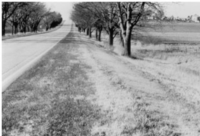
Figure 12. Typical Roadway with Roadside Hazard Rating Equal to 5.
