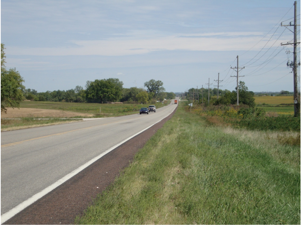
FIGURE 9 Photo of US-56 between Baldwin City and Edgerton, KS.
