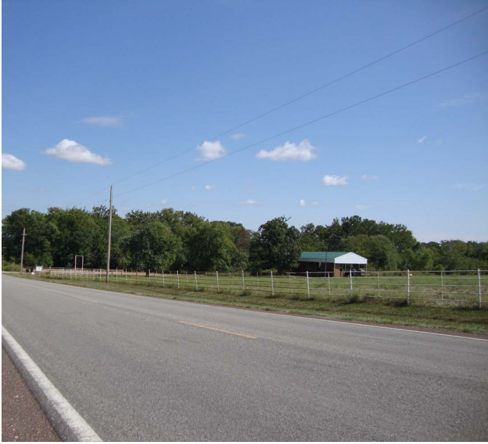
FIGURE 7 Photo of US-56, 1 mile west of Baldwin City.
