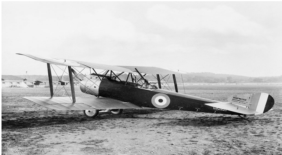
Sopwith 1 and 1/2 Strutter two-seater aircraft. This was the RFC's first aircraft to be equipped with a synchronization mechanism to allow the pilot to fire his machine-gun through the propeller arc. (IWM Q67507)
