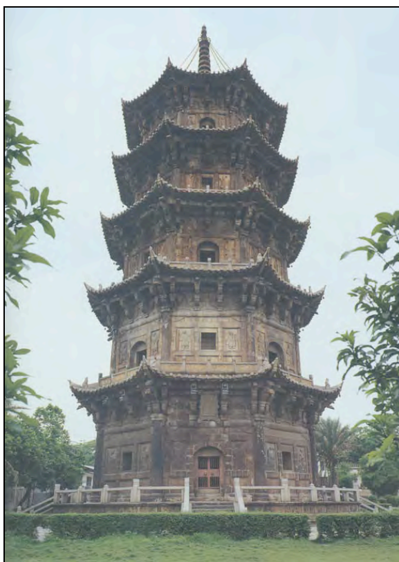
(Fig. II-33) West Pagoda, 1228–37. Southern Song, Kaiyuan si, Quanzhou, Fujian. Sekai bijutsu daizenshū , Tōyōhen 6, pl. 236.
