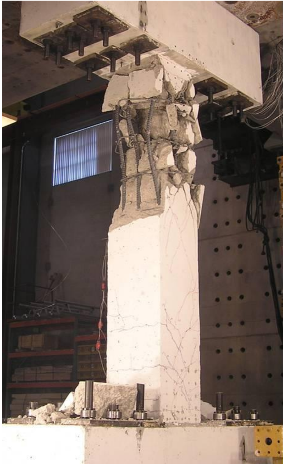
Figure 3.19: Final condition of Specimen 4.
