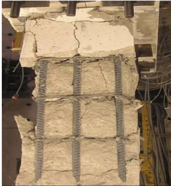
Figure 3.17: Crack pattern at the top of Specimen 4 for a maximum drift ratio of 2.5%.
