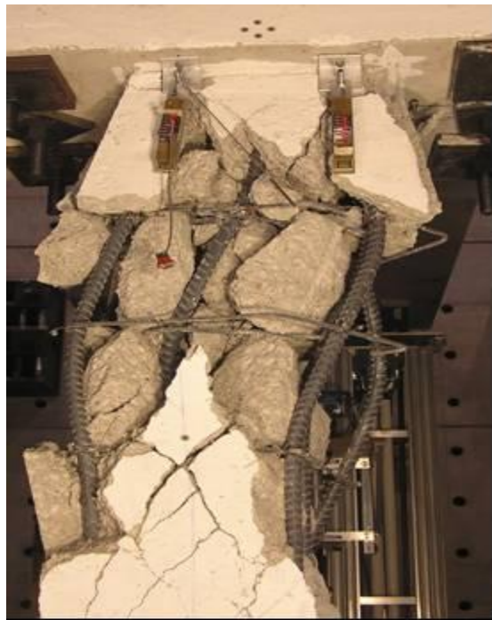
Figure 3.18: Condition of Specimen 4 for a maximum drift ratio of 3%. Damage to the concrete of the core and anchorage failure of the hoop caused buckling of the longitudinal reinforcement.
