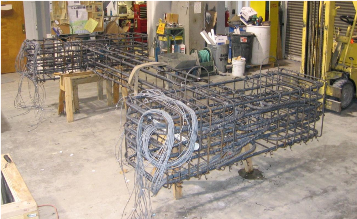
Figure 2.7: Specimen reinforcing cage
