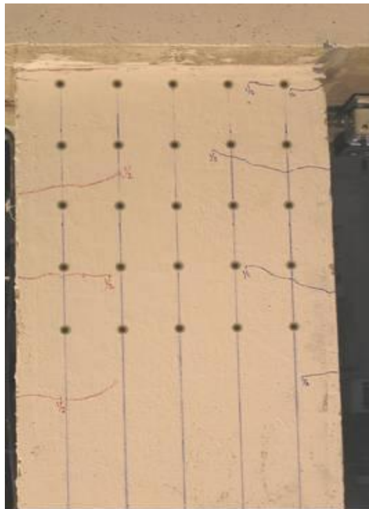
Figure 3.2: Crack pattern at top of Specimen 3 for maximum drift ratio of 0.50%.
