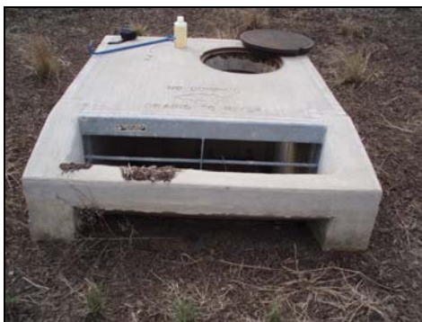
Photo 5. View of overflow structure at far end of bioretention basin close to Mize Lake.
