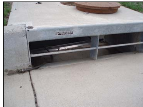
Photo 4. View of sewer from road and collection tube.
