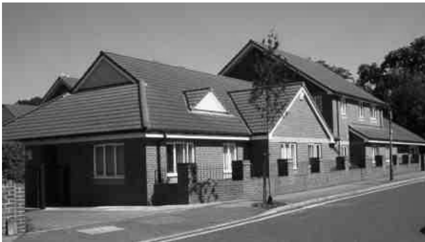
Figure 4.2: A Typical Surgery Building
