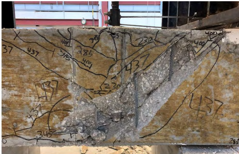
Figure 5.24 Anchorage failure observed in specimen 14-16E ( A_{tt}/A_{hs} = 0.551 )
