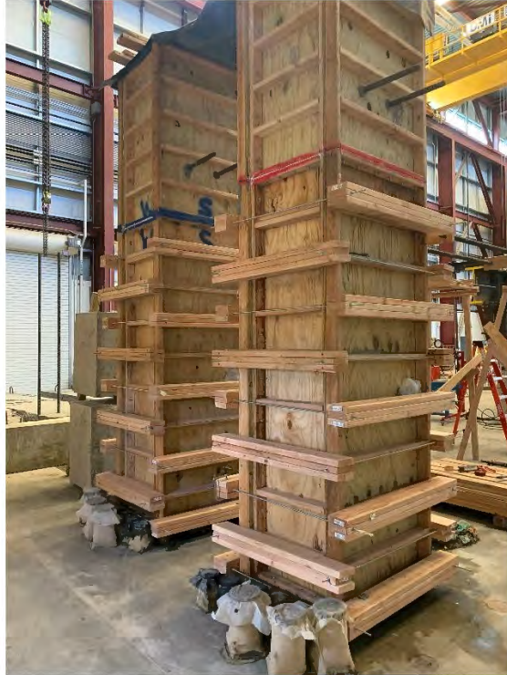
Figure 2.9 Clamping system to brace the vertical forms for No. 14 bar specimens
