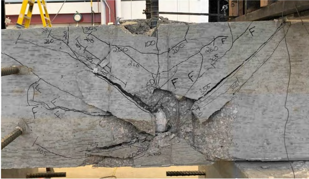
Figure 5.21 Anchorage failure observed in specimen 14-16C ( A_{tt}/A_{hs} = 0.356 ) tested under loading condition B
