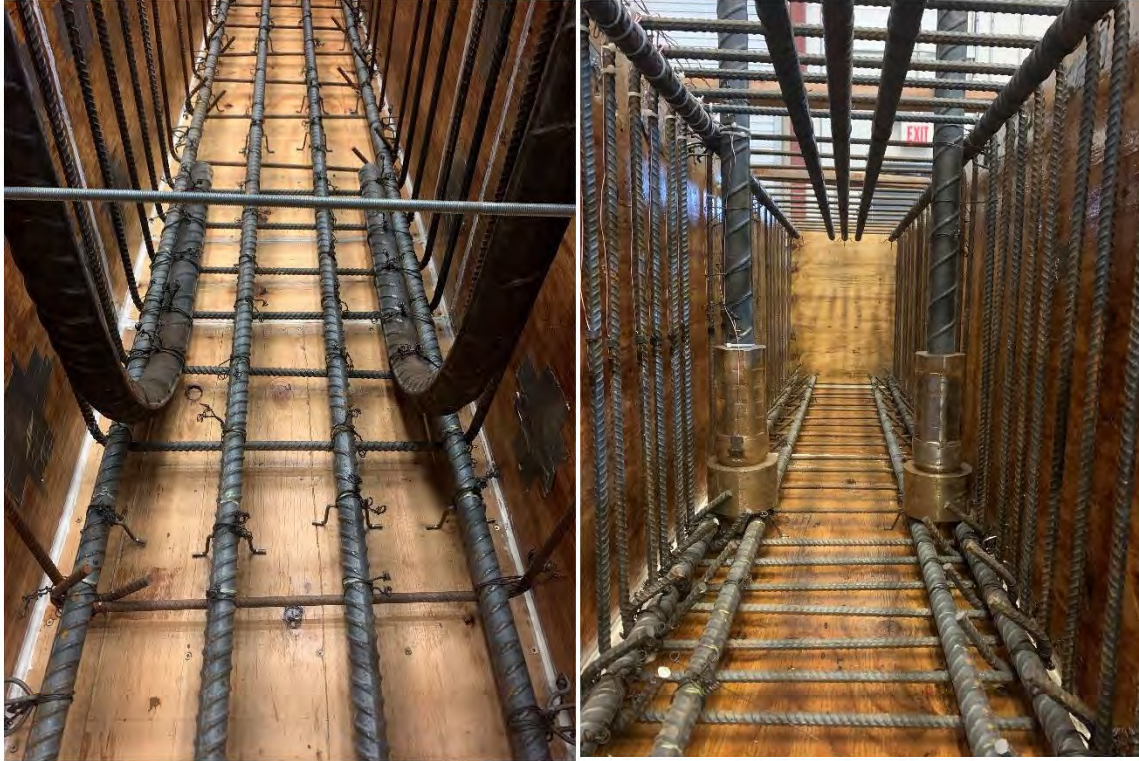
Figure 2.13 No. 18 hooked (left) and headed (right) bars tied to steel cages
