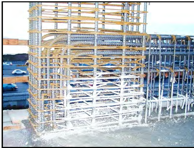
Figure 1.8 Steel congestion in an external beam-column joint caused by staggered hooked bars ( https://www.sefindia.org )
