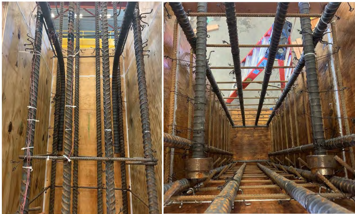
Figure 2.12 No. 14 hooked (left) and headed (right) bars tied to steel cages
