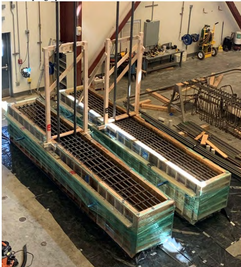
Figure 2.10 Horizontal formwork for No. 18 bar specimens
