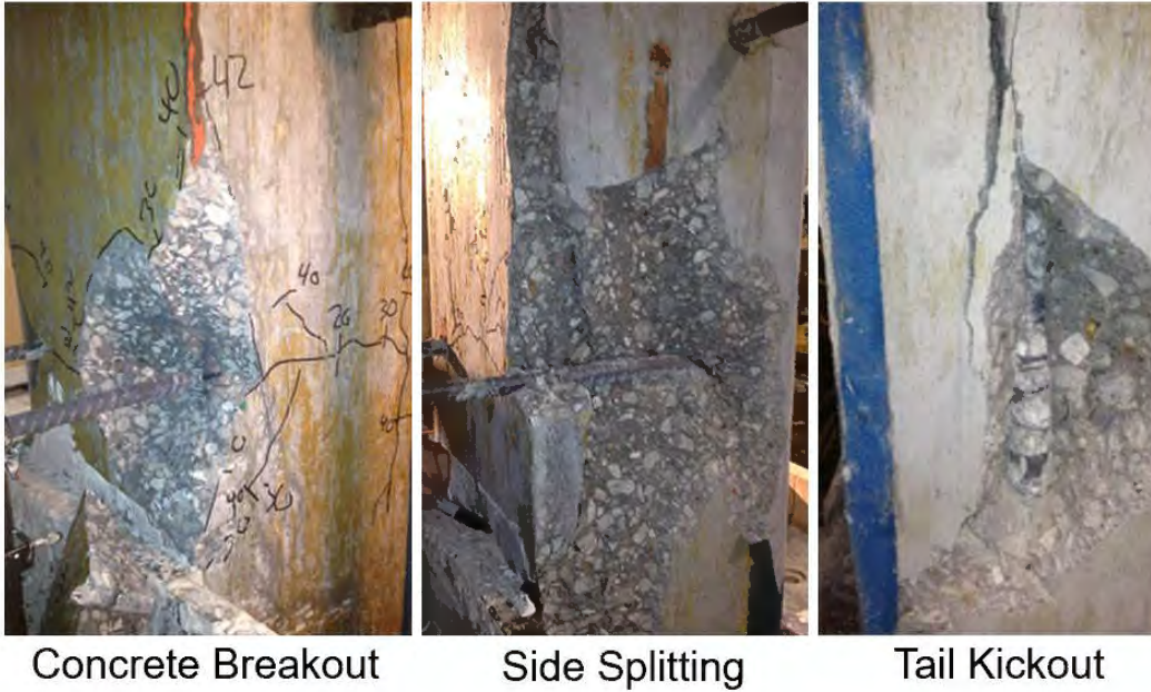
Figure 1.7 Primary failure modes observed in hooked bar specimens (Sperry et al. 2015b)
