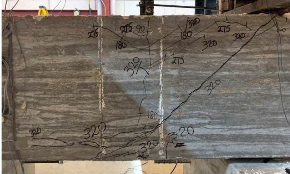
Figure 5.18 Shear-like failure observed in specimen 14-1A ( A_{tt}/A_{hs} = 0 ) tested under loading condition B
