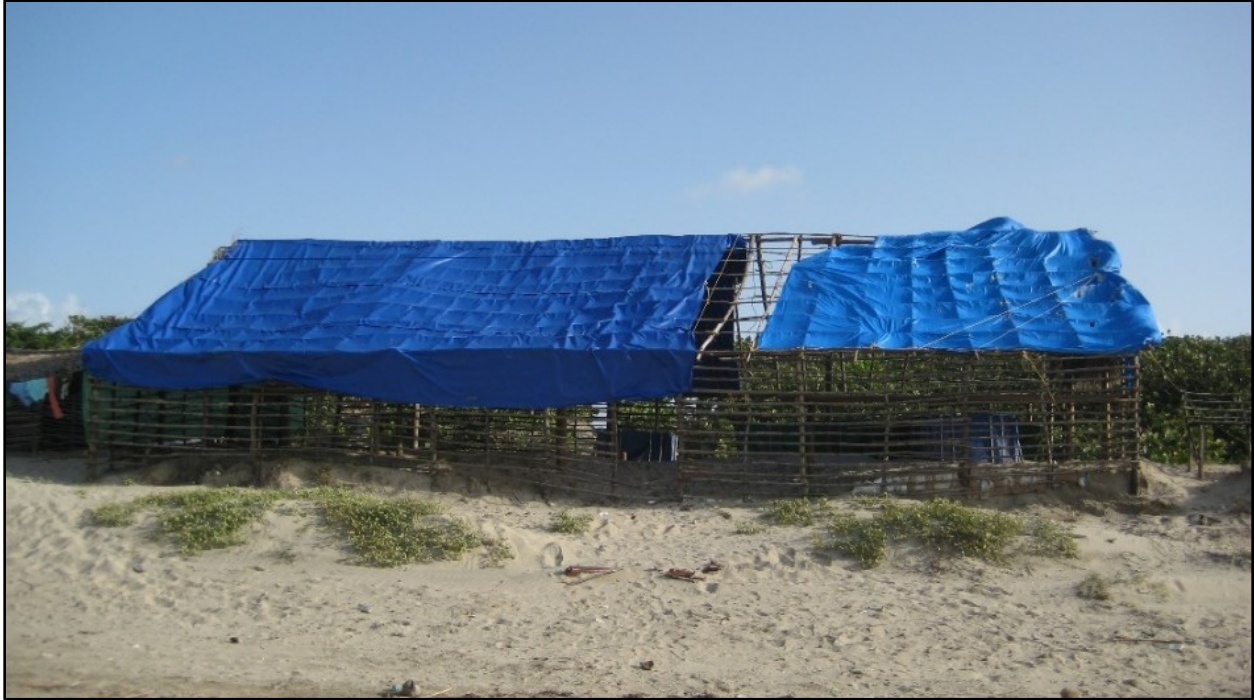
Figure 18: A Rudimentary JPF near Kaukira, Gracias a Dios, Honduras. Instead of concrete basins, builder's lumber, and a metal roof, this JPF uses plastic basins, a low grade 'stick' frame, and a tarp roof. Such a set-up is not designed to last long, but it is cheap to build for a processor concerned with reducing their upfront investment and risk. (Source: Author, 2014).
