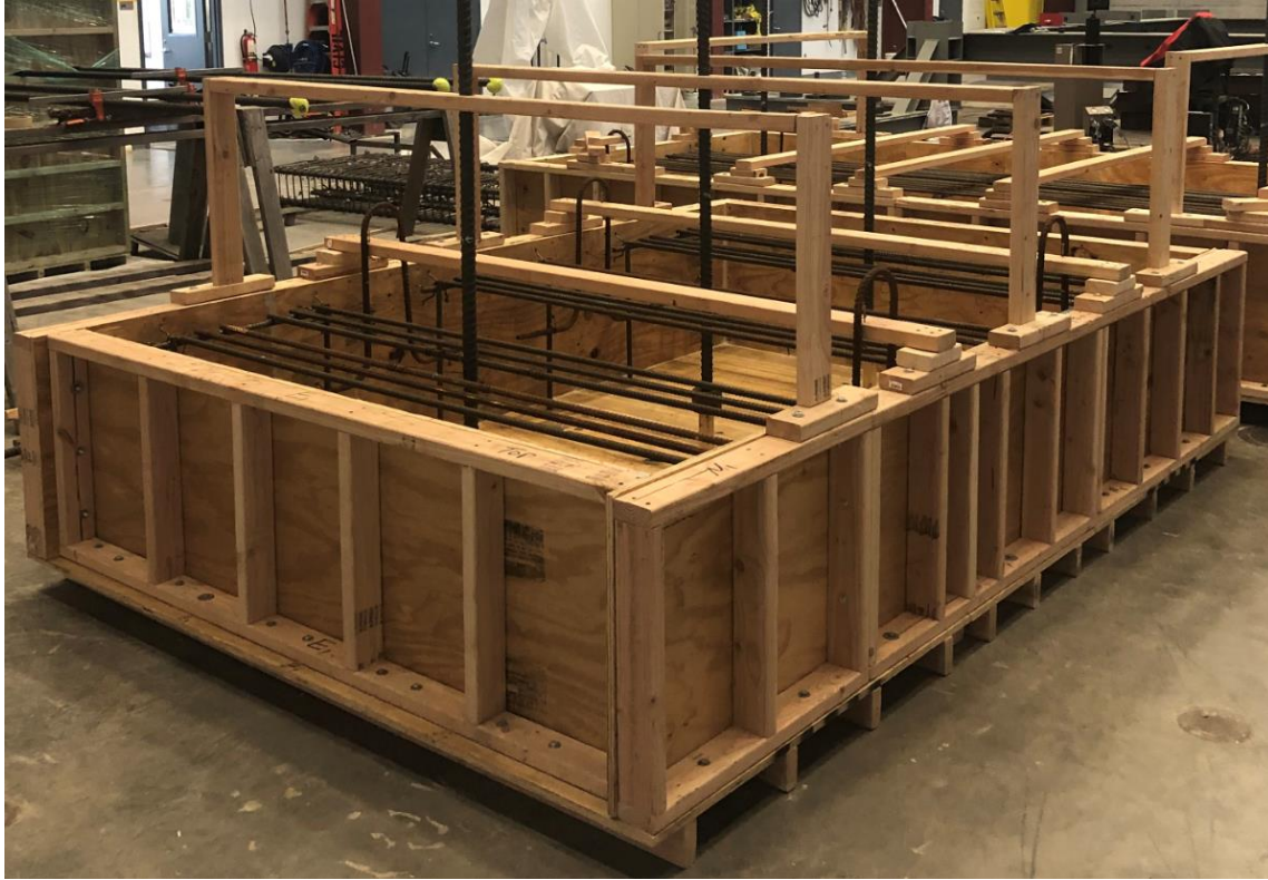
Figure 2.12 Slab specimen formwork
