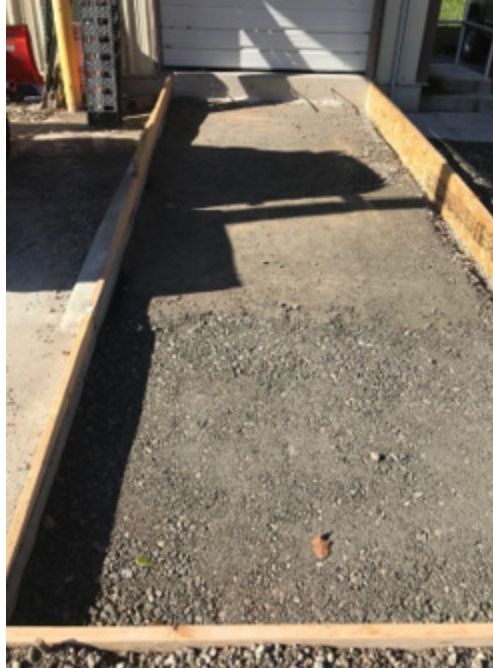
Figure 4.41: The qualification slab for KS-IC-LC-HPC-1 prior to placement
