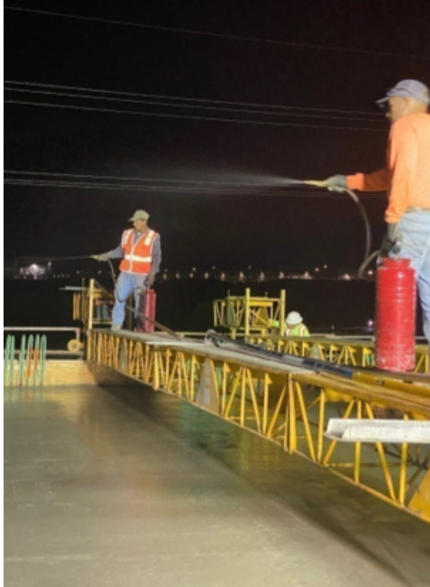
Figure 4.66: Applying finishing aid to the concrete surface
