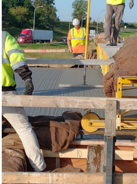
Figure 4.30: Tining the deck before the application of curing compound
