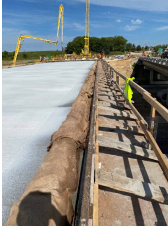
Figure 4.32: Burlap placement on the barrier reinforcement
