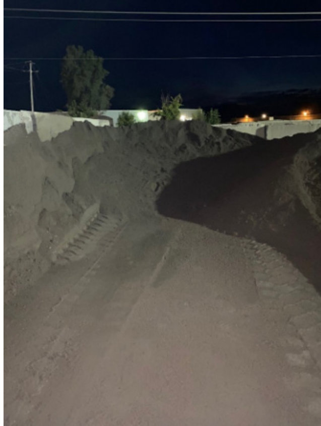
Figure 4.34: Disturbance of the bottom of the stockpile
