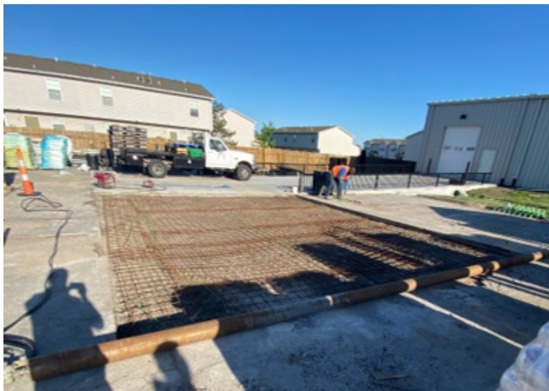
Figure 4.62: The qualification slab for KS-IC-LC-HPC-3
