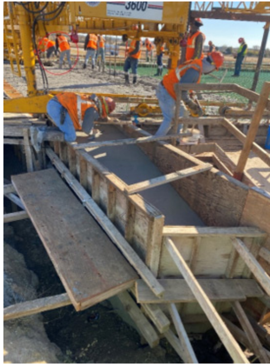
Figure 4.51: Walking observed on freshly consolidated concrete
