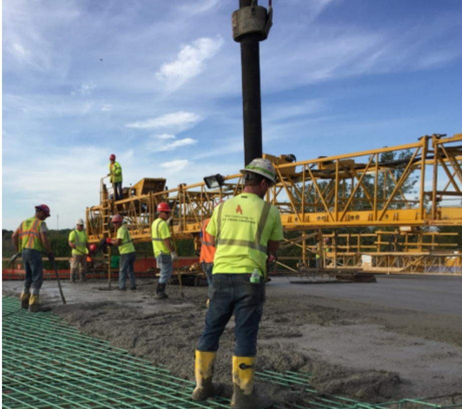
Figure 4.16: Placing, consolidation, and finishing equipment
