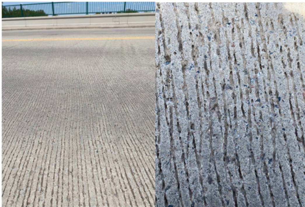
Figure 5.20: Poorly tining of MN-IC-LC-HPC-6 (a) an overview; (b) a close-up view
