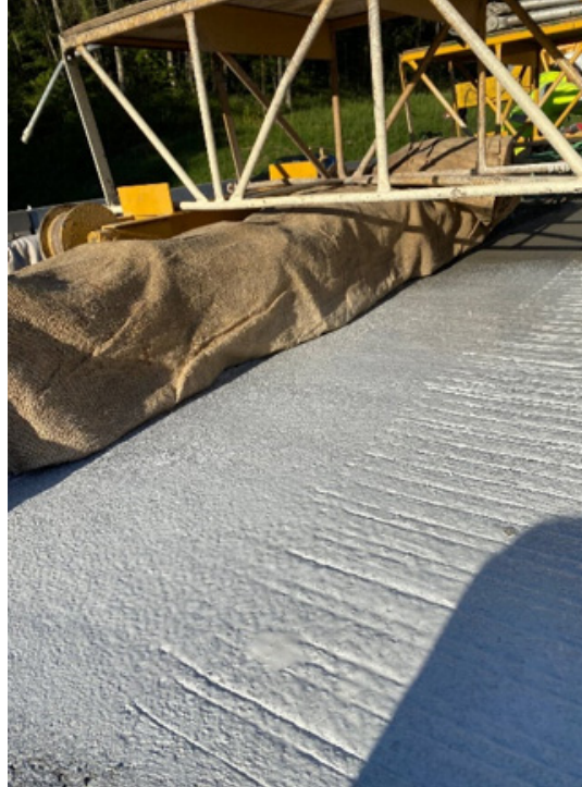
Figure 4.37: Burlap placement on the barrier reinforcement
