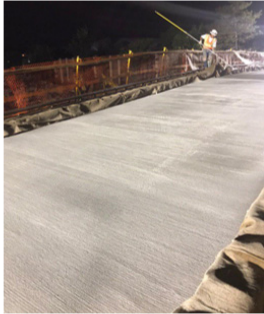
Figure 4.14: Burlap placement on the barrier reinforcement
