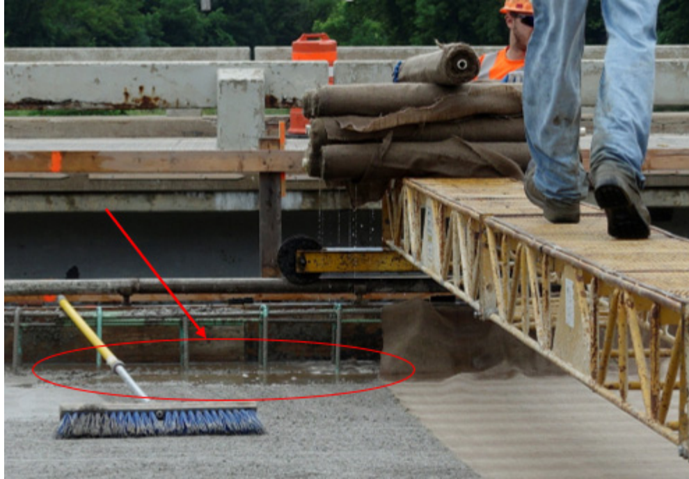
Figure 4.3: Water from burlap dripping onto the deck
