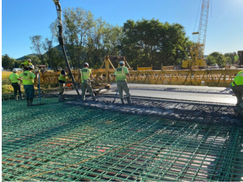
Figure 4.35: MN-IC-LC-HPC-9 placement
