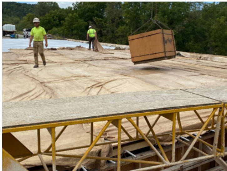
Figure 4.39: Wet curing application on MN-IC-LC-HPC-9
