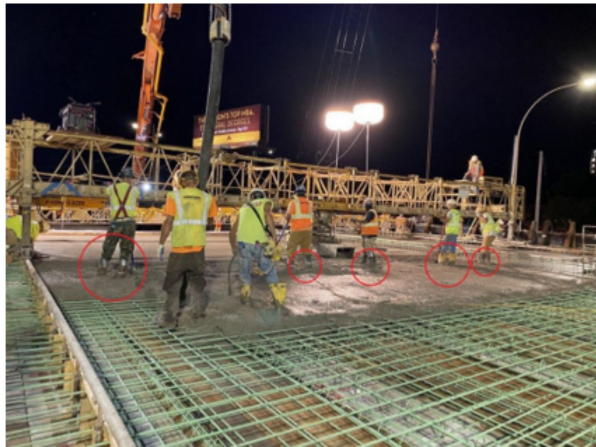
Figure 4.22: Walking observed on freshly consolidated concrete
