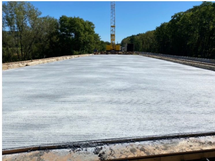
Figure 4.36: Application of the curing compound on the deck
