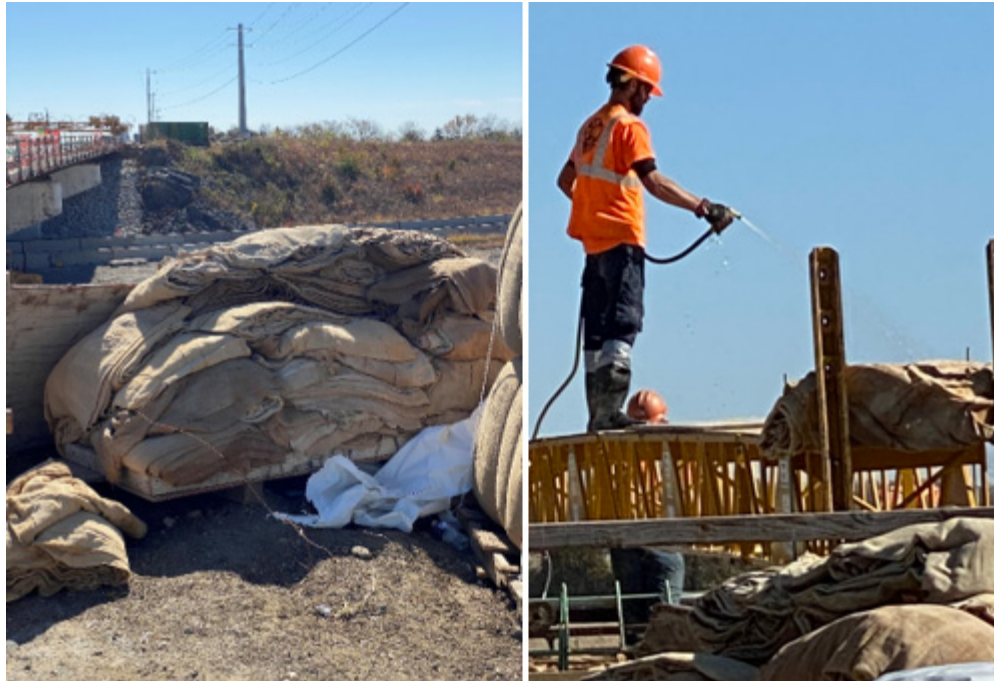
Figure 4.54: Burlap placement of KS-IC-LC-HPC-2 (a) dry burlap; (b) wetting the burlap on the deck
