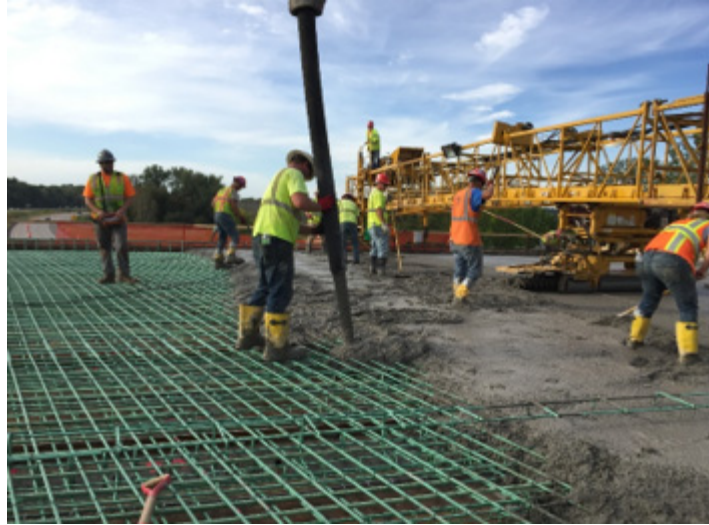
Figure 4.17: Walking through consolidated concrete
