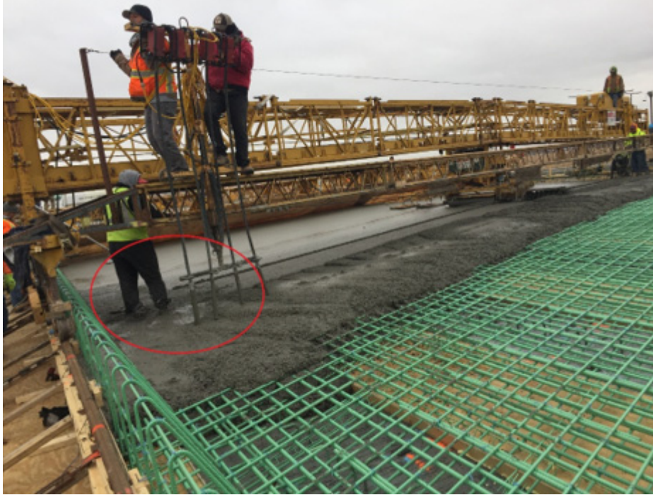
Figure 4.46: Walking through consolidated concrete
