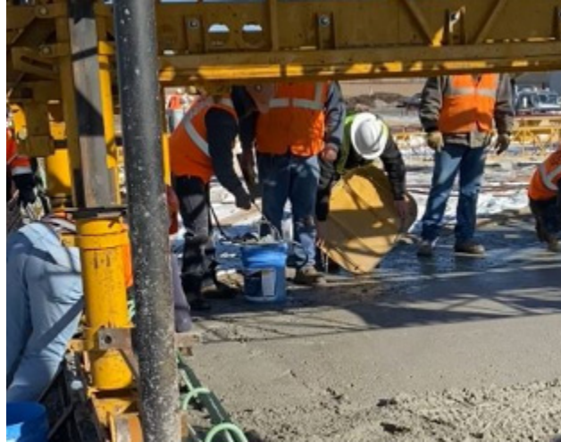
Figure 4.58: Applying finishing aid to the concrete surface
