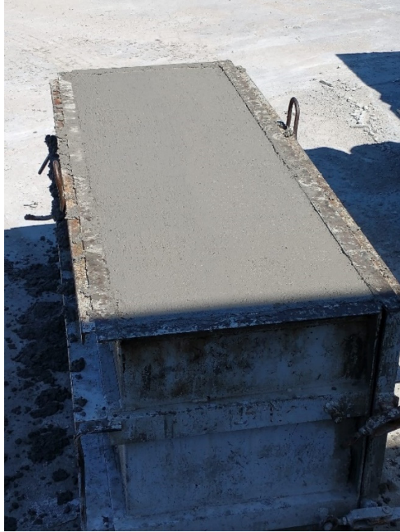
Figure 4.26: Placement of second truckload in second trial placement (containing set retarding admixture) with no observable air pockets on the concrete surface
