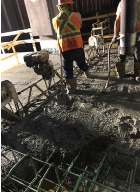
Figure 4.9: Placement, consolidation, and finishing of MN-IC-LC-HPC-5
