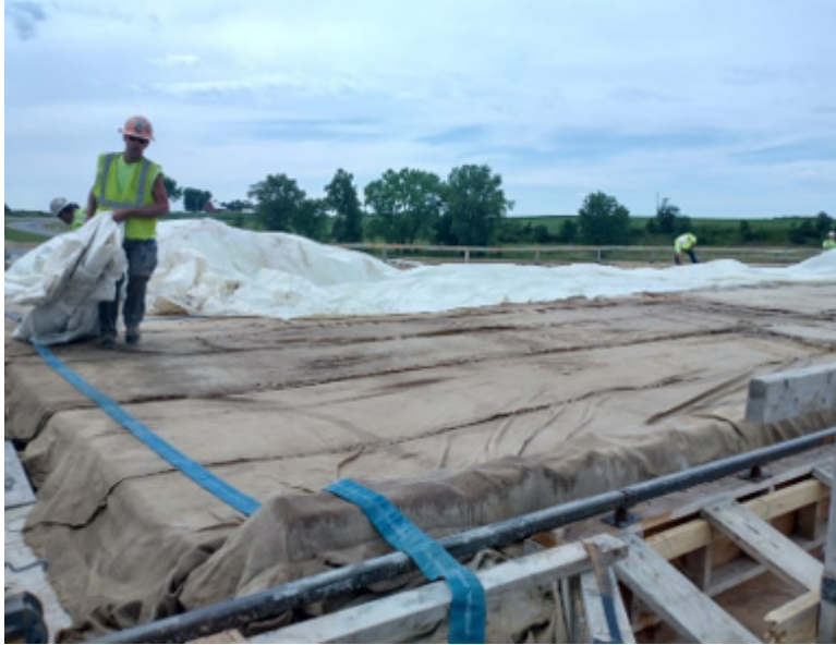
Figure 4.33: Covering the deck with wet burlap and plastic sheeting
