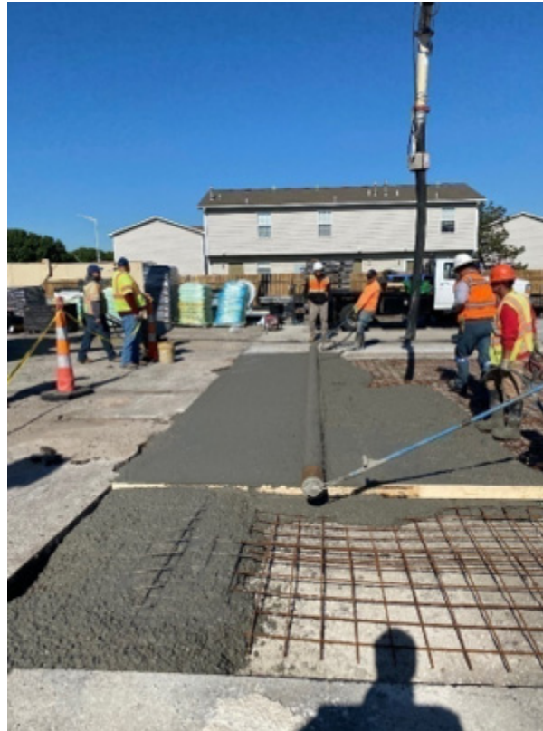
Figure 4.63: The qualification slab placement equipment
