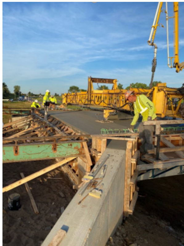
Figure 4.28: Finishing equipment
