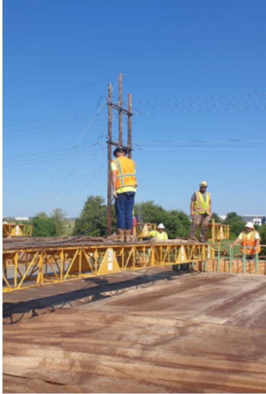
Figure 4.68: Rewetting the burlap on the deck
