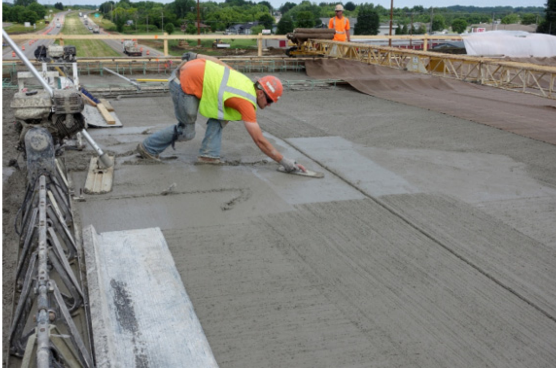
Figure 4.4: Walking through freshly consolidated concrete
