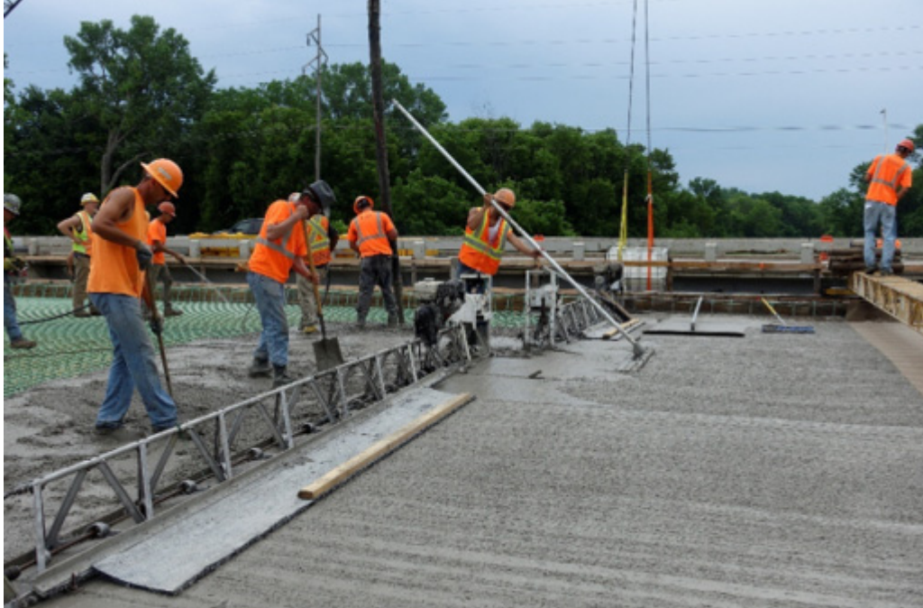
Figure 4.2: Finishing equipment for MN-IC-LC-HPC-2 subdeck
