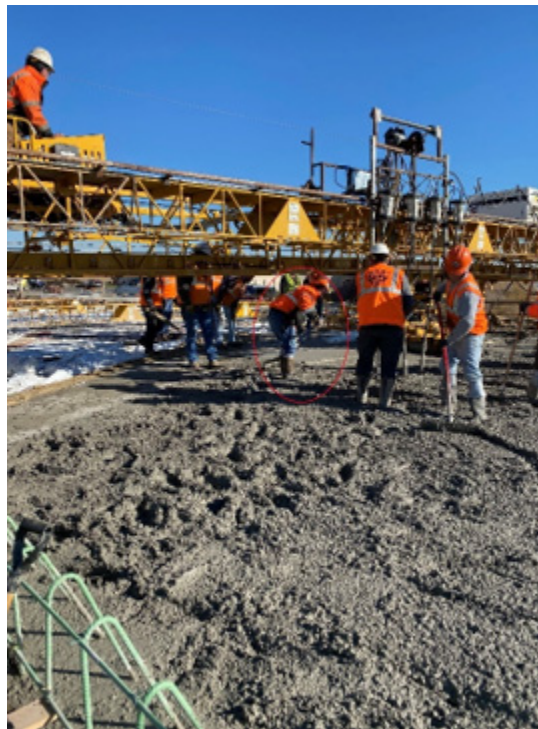
Figure 4.56: Walking observed on freshly consolidated concrete
