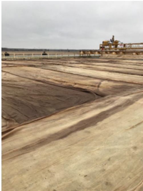
Figure 4.48: Burlap placement on the deck
