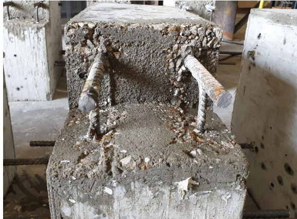
Figure 2.16: Exposed Aggregate Look of Base Blocks
