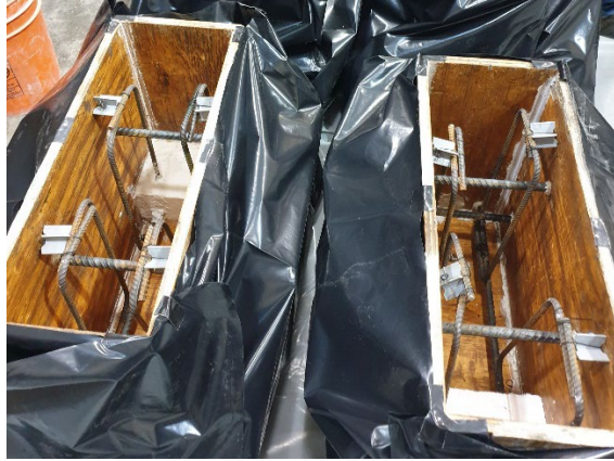
Figure 2.15: Base Blocks Formwork
