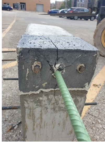
Figure 3.4: Splitting Cracks on Beam-End Specimen
