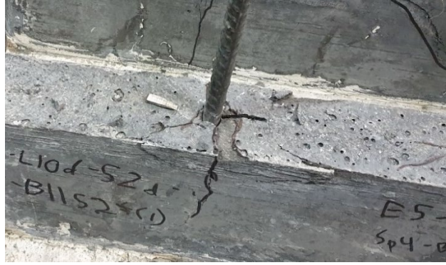
Figure 3.2: Splitting Cracks on Pullout Specimen
