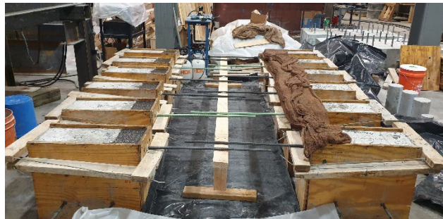
Figure 2.17: UHPC Bond Block Formwork
