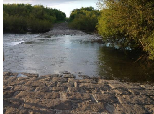
Photo 6. Flooded historical low water crossing in the Guichón vicinity. Photo by Dr. Carol Baldwin.
