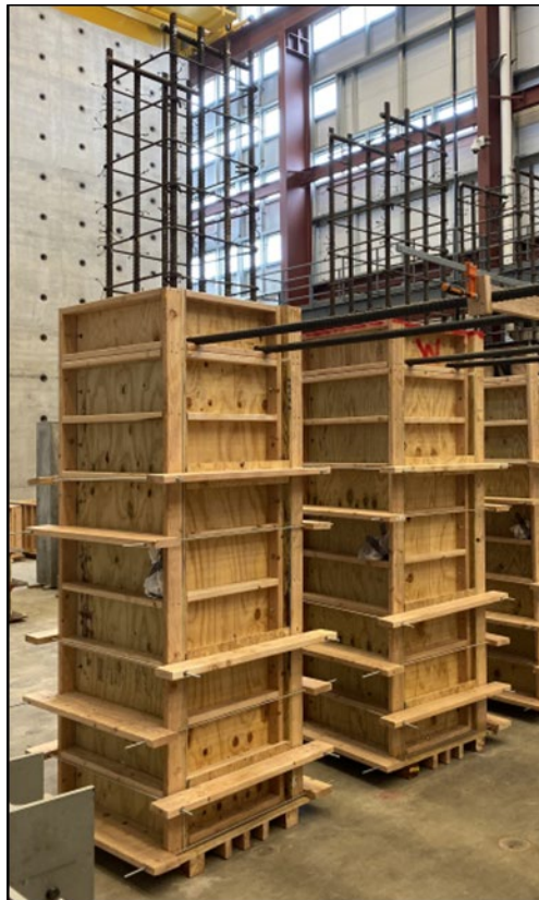
Figure 12 - Formwork for the No. 14 bar specimens
