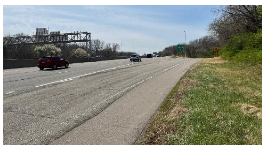
Figure 19: Facing southbound direction near RP 357.7.
