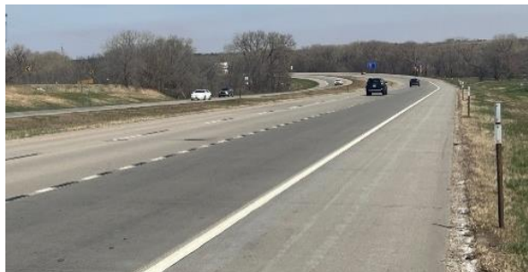
Figure 15: Facing eastbound direction near RP 295.2.
