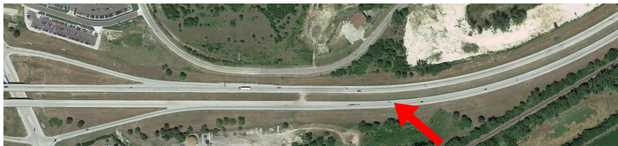
Figure 21: RP 295.4 location with superelevated transition noted.
