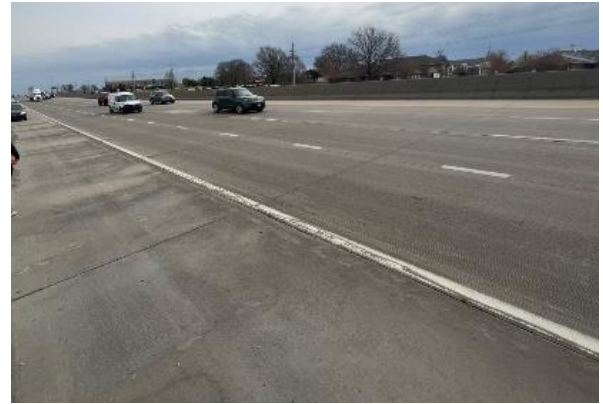
Figure 12: Facing northbound direction near RP 217.55.
