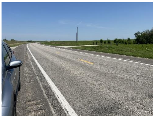
Figure 18: Facing eastbound direction near RP 330.1.
