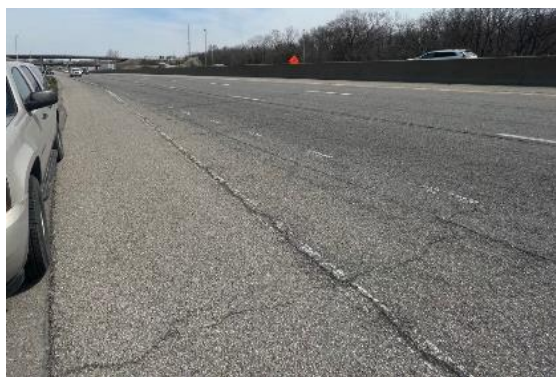
Figure 20: Facing northbound direction near RP 357.7.
