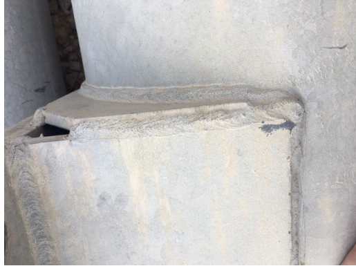
Figure 3.8. Gusseted Box Connection Welding: a) Donated Structure 165 and b) Test Specimen
