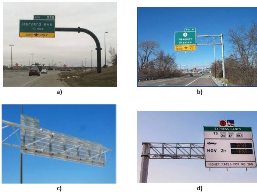
Figure 1.1. COSS Construction Types: a) monotube; b) two mast-arms; c) three mast-arms; d) four mast-arms (Senior 2018)
