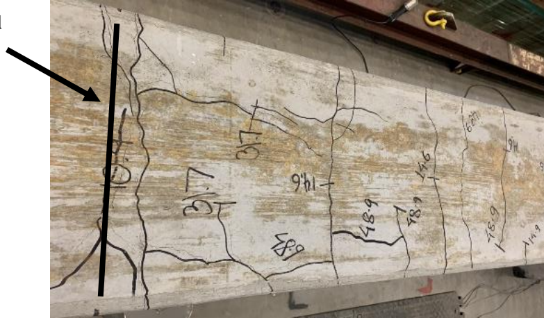
Figure 4.5: Parallel-splitting cracking (14-f)
