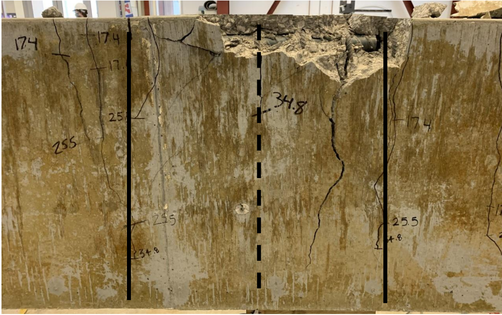
Figure E.5: Photo of 14-e after failure
