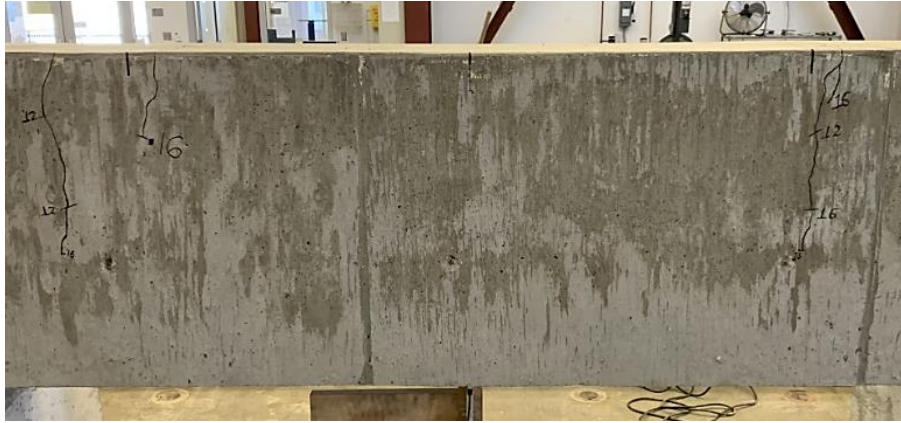
(a) Initial cracking
