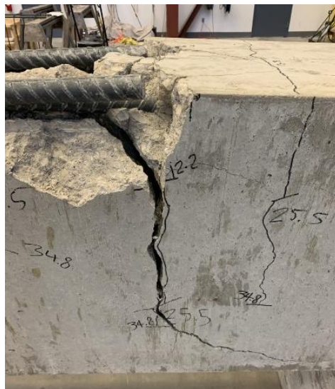
Figure 4.6: Unconfined lap splice failure (14-a)
