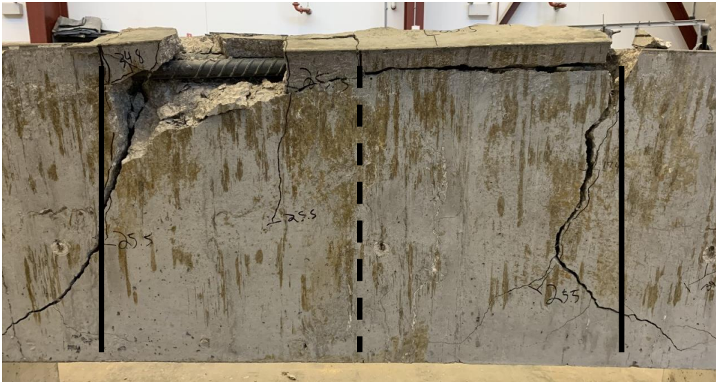
Figure E.4: Photo of 14-d after failure
