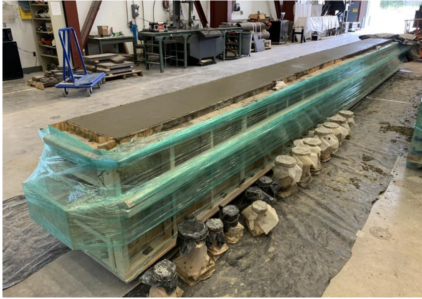
Figure 3.8: Formwork after concrete placement (14-b)
