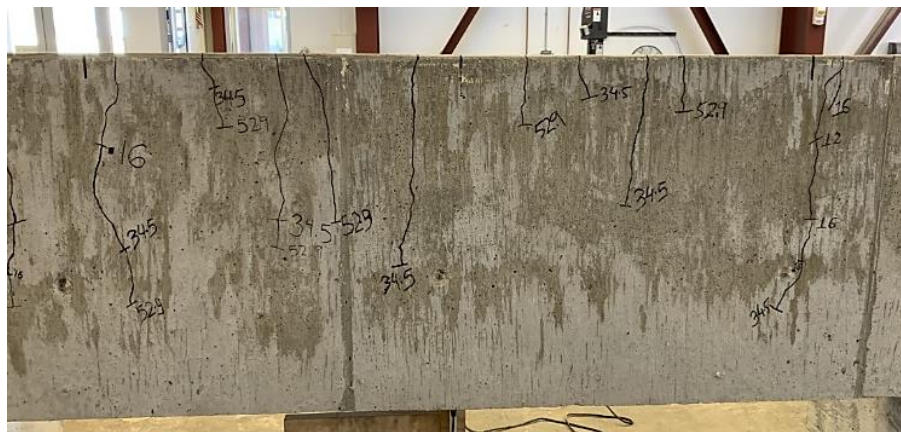
(b) Cracking during increased loading
