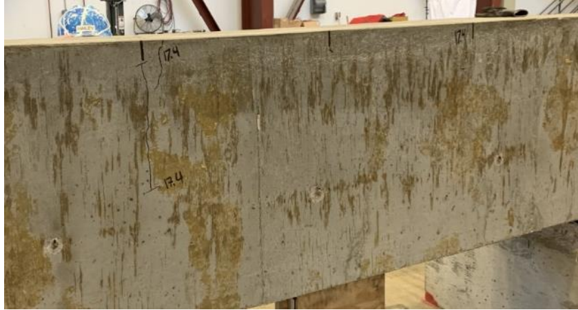
(a) Initial cracking
