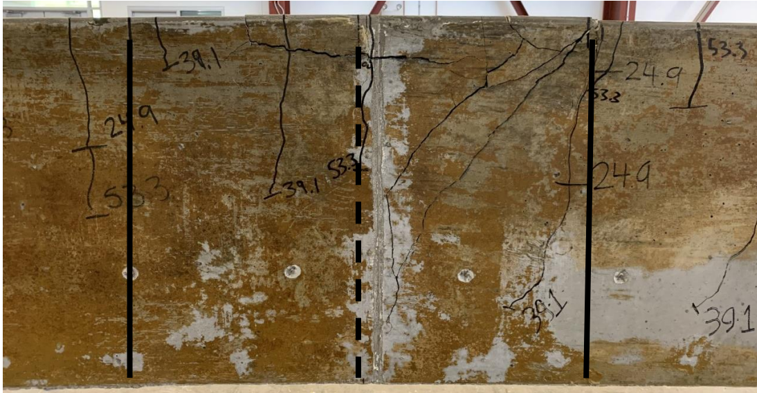
Figure E.11: Photo of 18-d after failure
