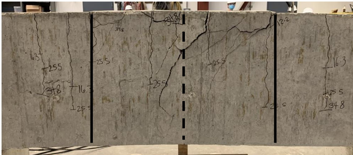
Figure E.2: Photo of 14-b after failure
