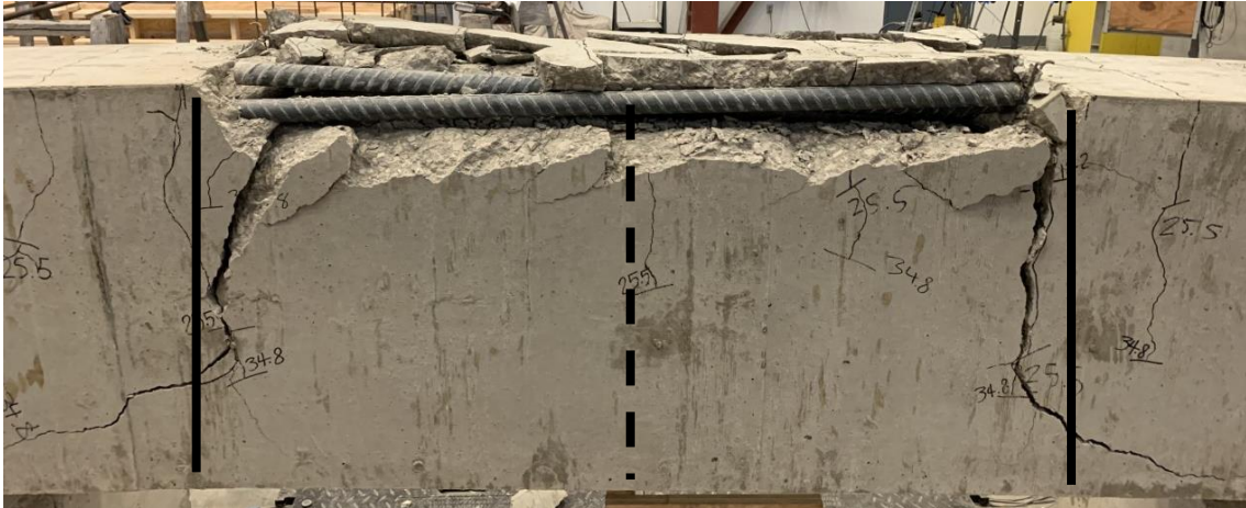
Figure E.1: Photo of 14-a after failure
