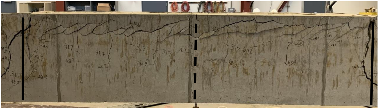
Figure E.6: Photo of 14-f after failure
