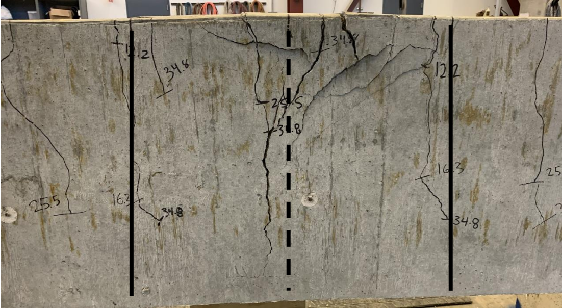
Figure E.3: Photo of 14-c after failure
