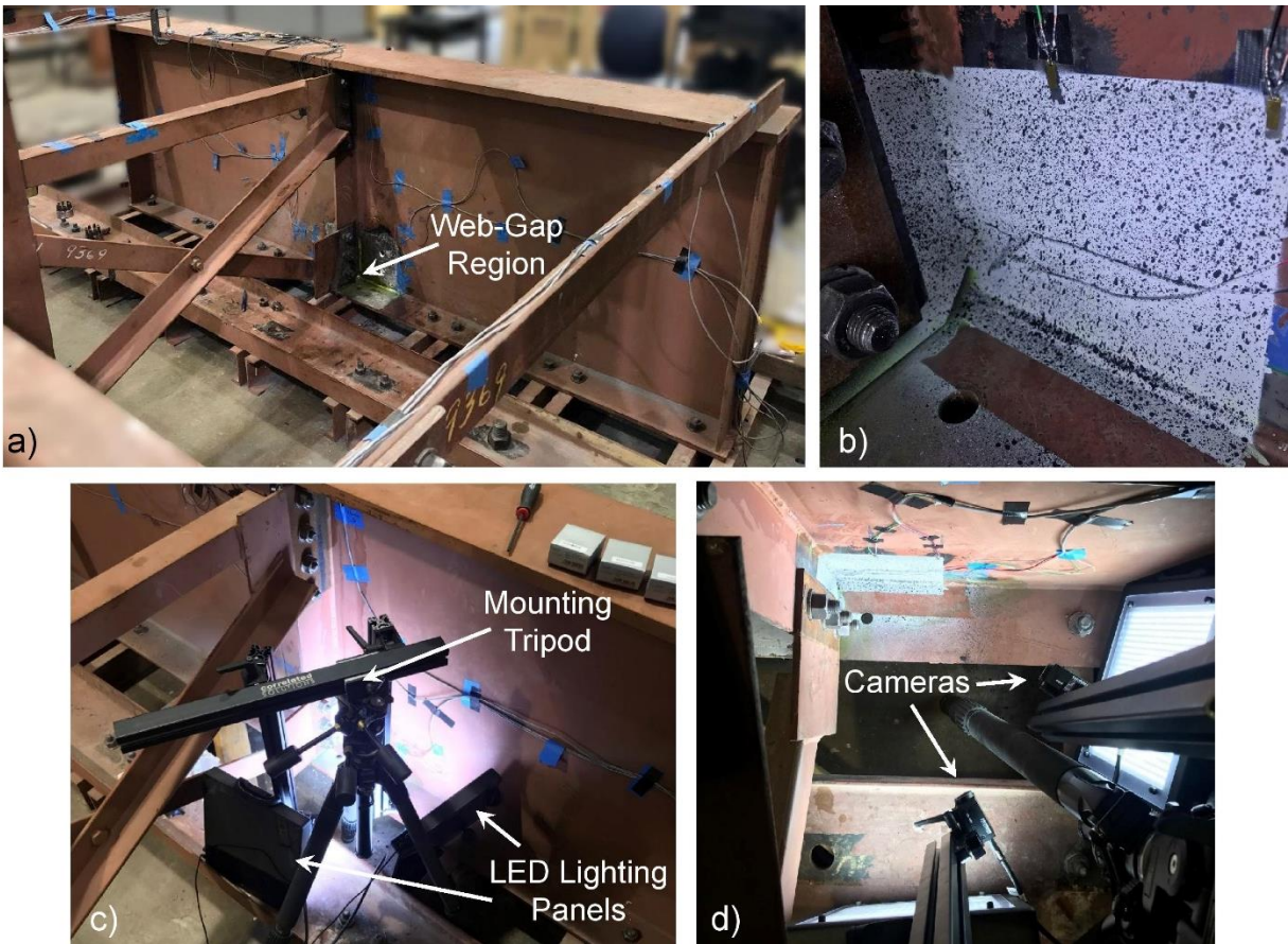
Figure 10. (a) Distortion-induced fatigue test frame; (b) applied high-contrast surface pattern in the web-gap region; (c) DIC hardware placement; and (d) detailed orientation of DIC hardware seen from above.
