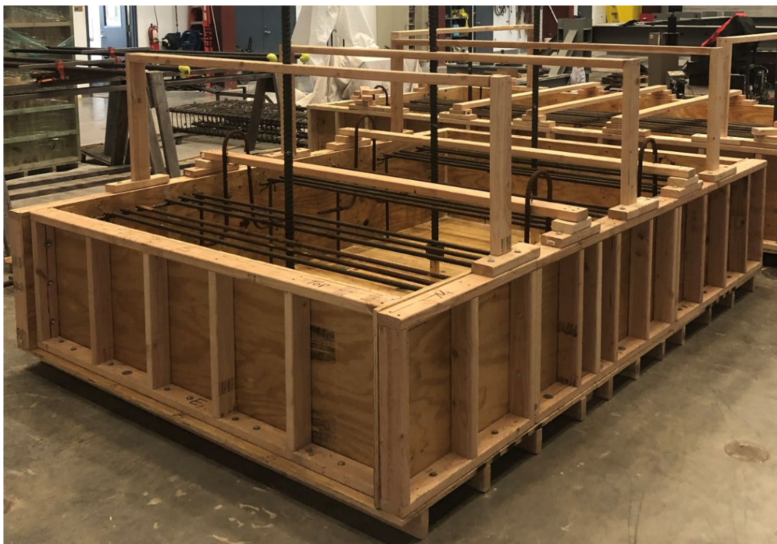
Figure 2.12 Slab specimen formwork
