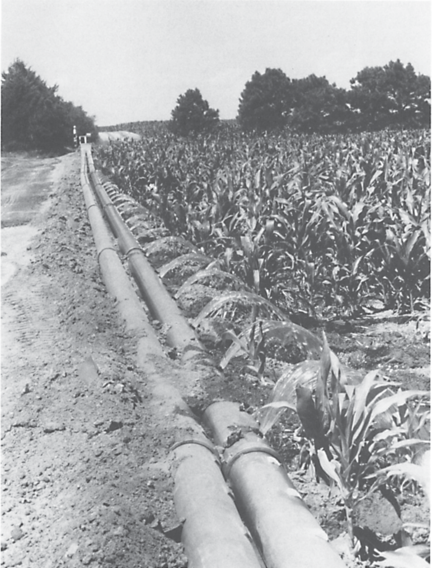
Cablegation sequentially opens gates in order to flood furrows. Chase County, Nebraska.
