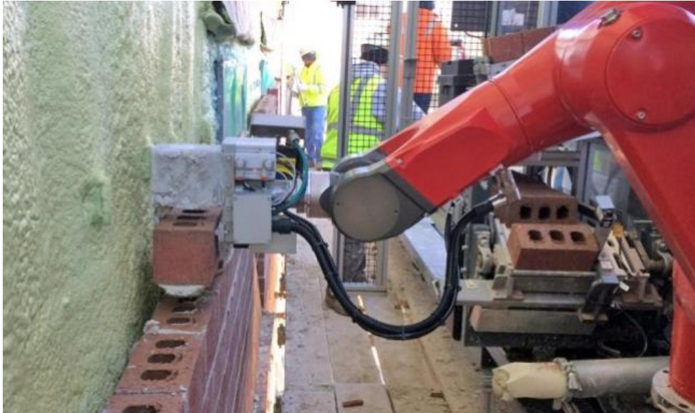
FIGURE 2.11 SAM bricklaying robot (Construction Robotics 2018)
