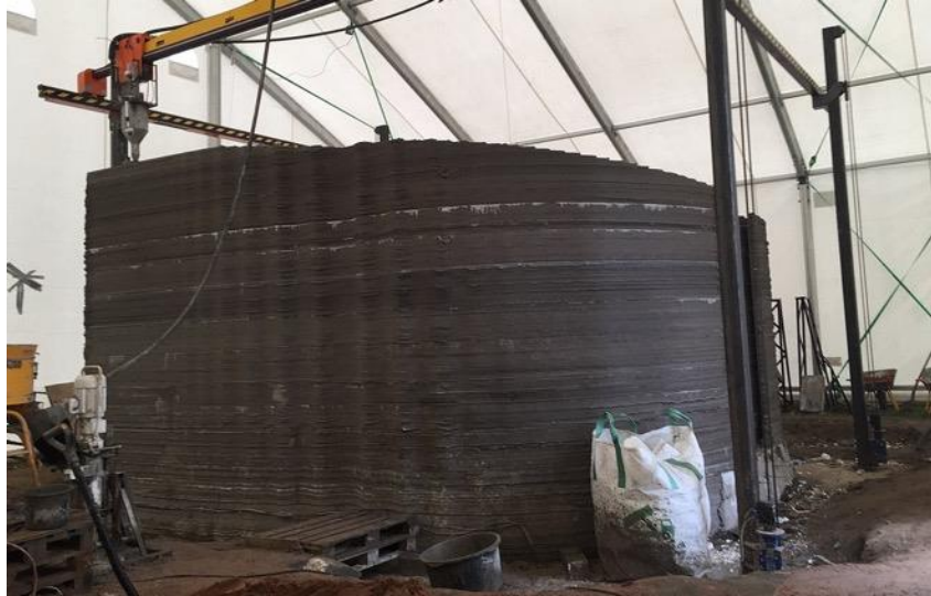
FIGURE 2.13 3D printed walls (3D Printhuset, 2018)
