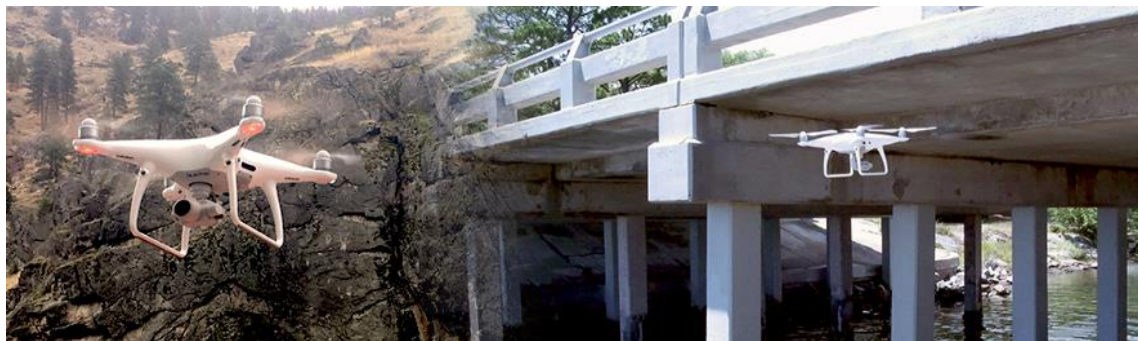
FIGURE 2.15 UAV application for highway construction (FHWA 2018)
