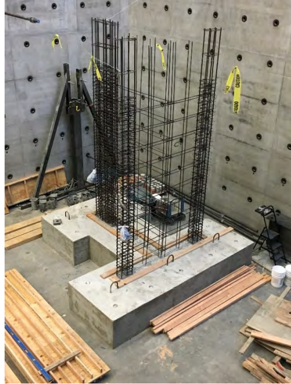
(b) Lift 1 steel cage
