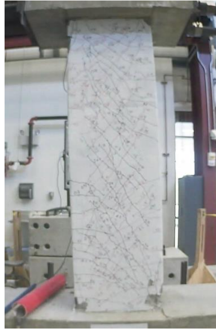
Figure C.49 – D80-3.5 at -2% chord rotation, second cycle
