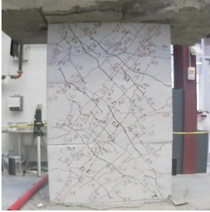
Figure C.9 – D100-1.5 at +2% chord rotation, second cycle
