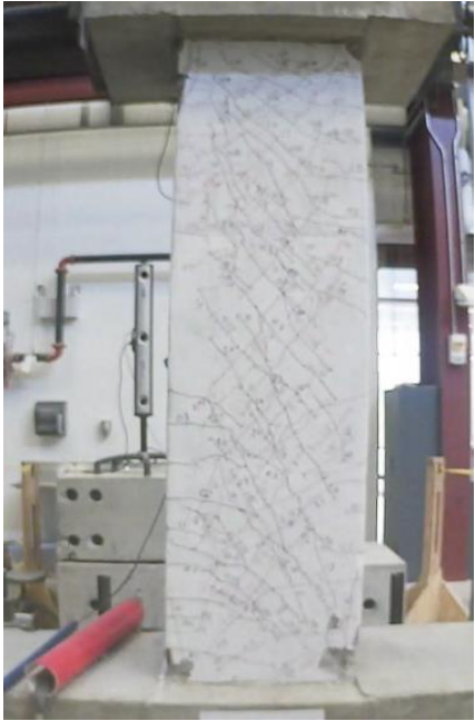
Figure C.48 – D80-3.5 at +2% chord rotation, second cycle
