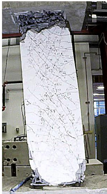
Figure C.75 – D120-3.5 at -8% chord rotation, second cycle
