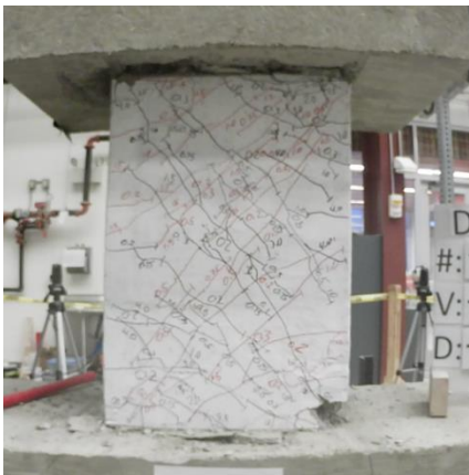
Figure C.3 – D80-1.5 at +4% chord rotation, second cycle
