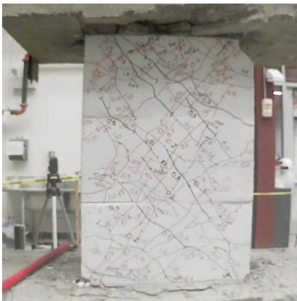
Figure C.11 – D100-1.5 at +4% chord rotation, second cycle
