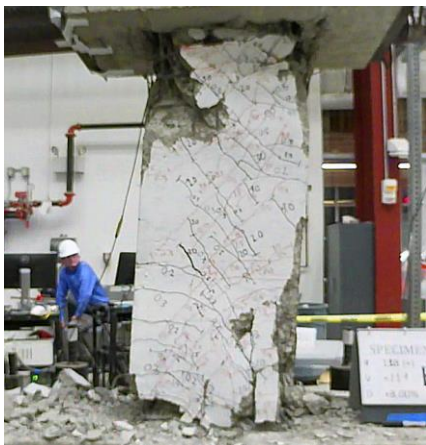
Figure C.28 – D80-2.5 at +8% chord rotation, second cycle
