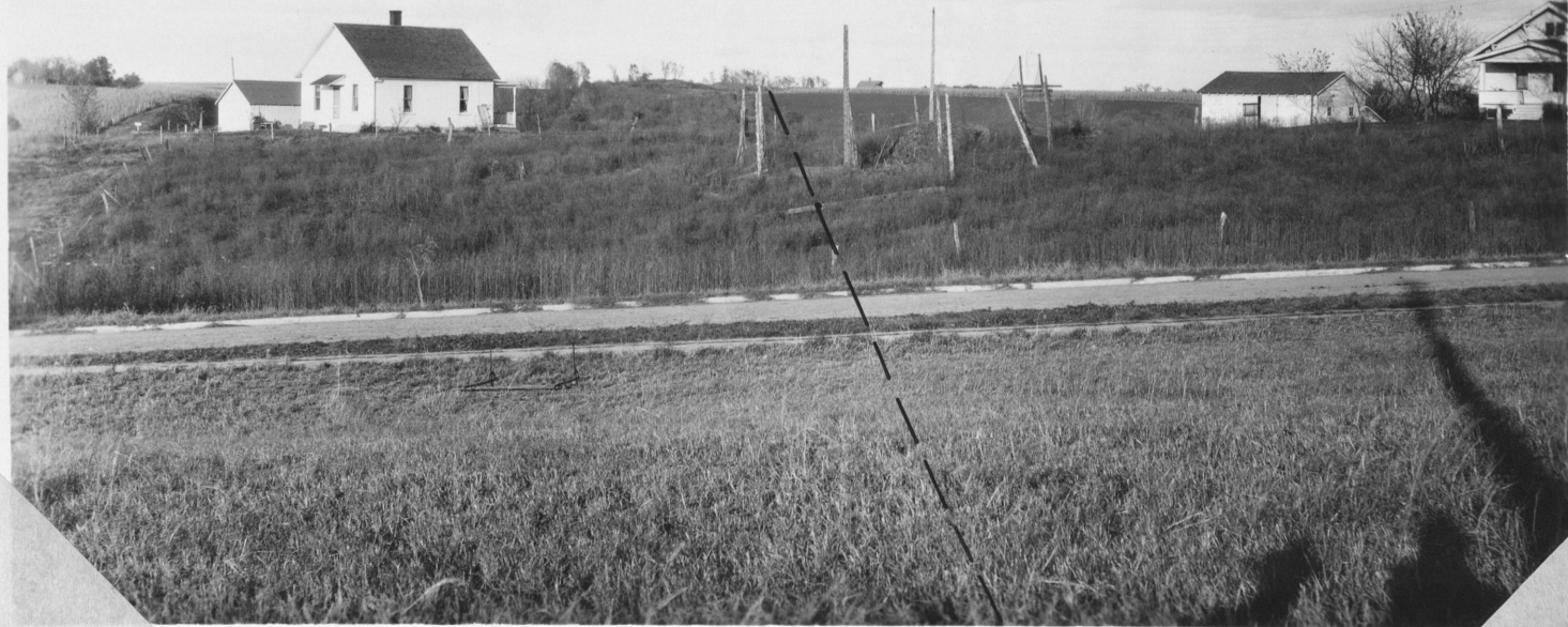
View No. 11 Line A Photo shows location of Line A crossing the paved street (Burnes Street in Gretna).
