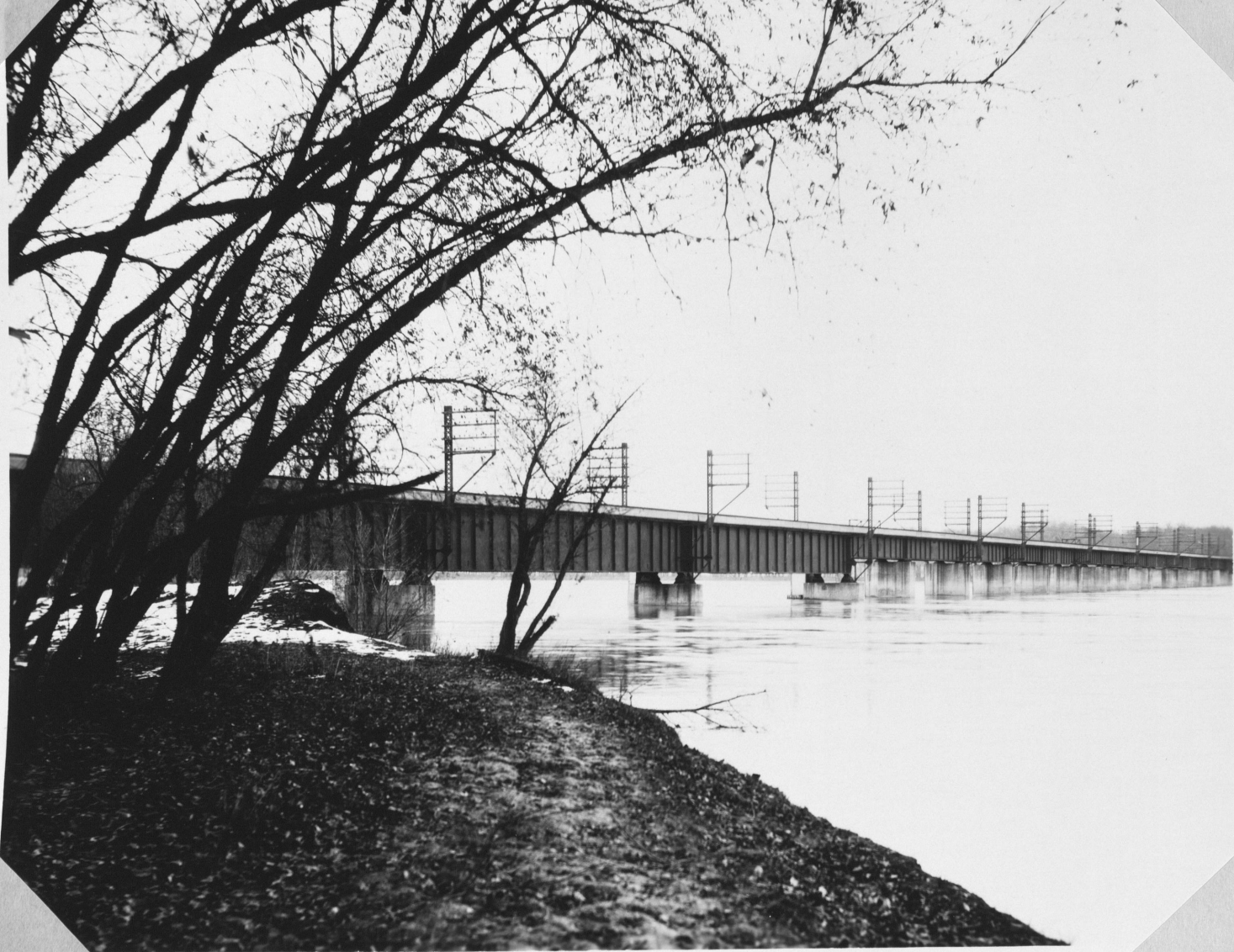
View No. 8 Line A Burlington Railroad-Platte River Bridge. Line A bridge is directly below this bridge. Line B bridge above the same.
