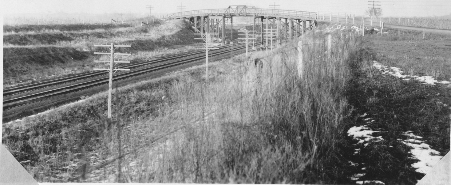
View No. 14 Lines B-C Present overhead structure southwest of Ashland on present road.
