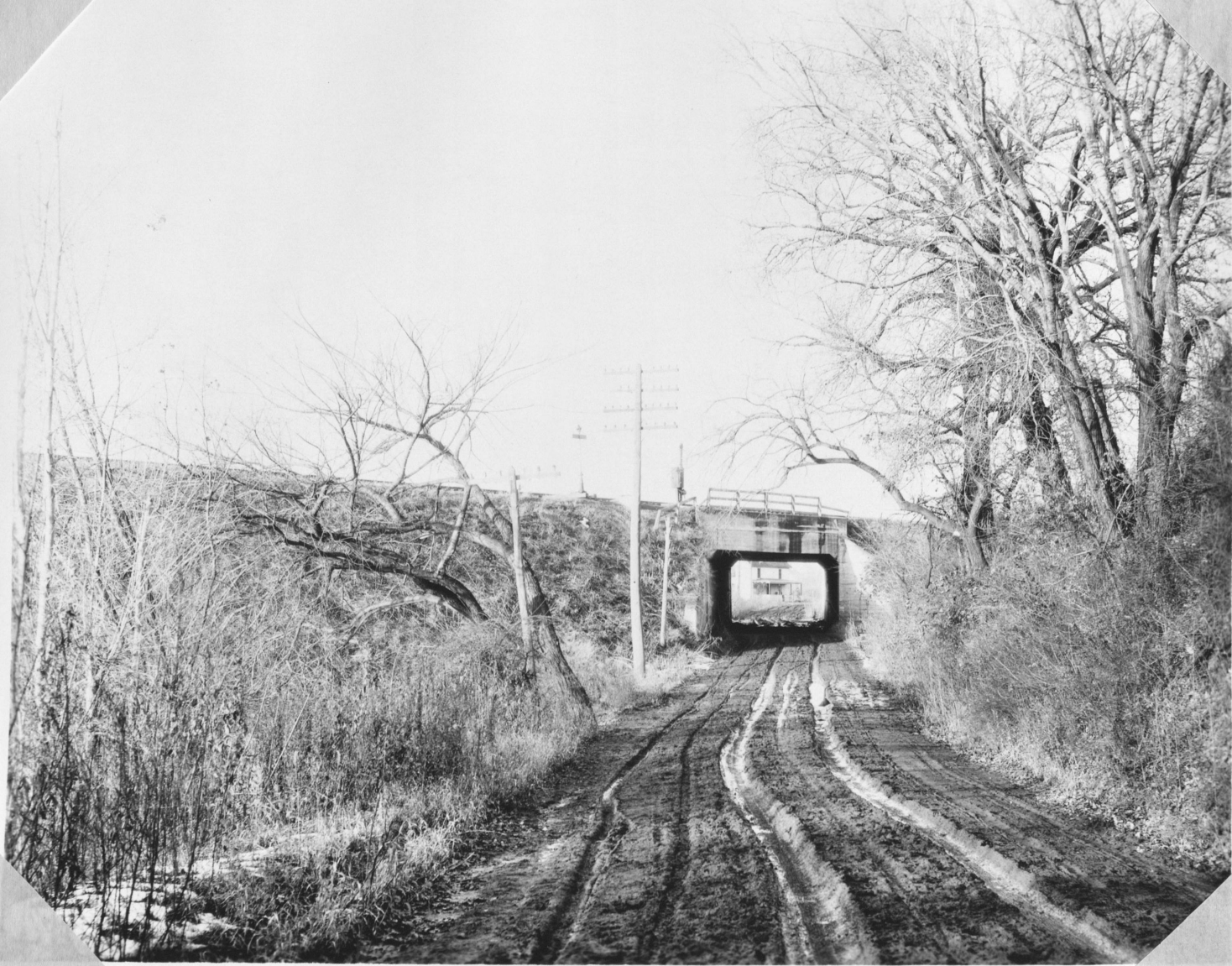
View No. 6-A Underpass in place north of Sta. 934 on present road via Salt Creek Bridge and 13th St. to Ashland.
