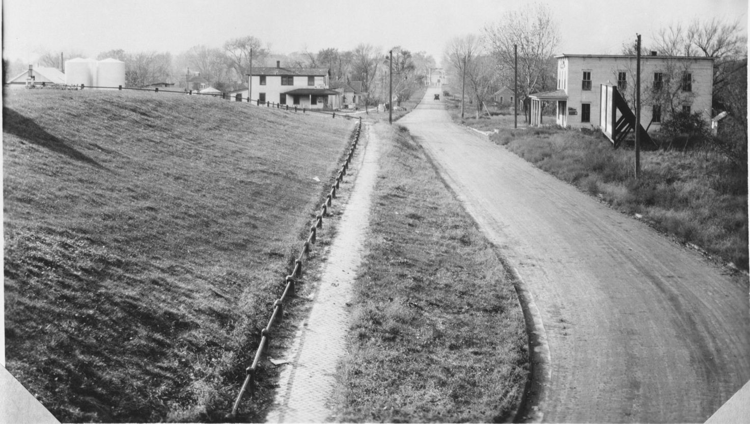
View No. 4 Line A Silver Street in Ashland. Looking west from top of overpass (#5) Sta. 984.
