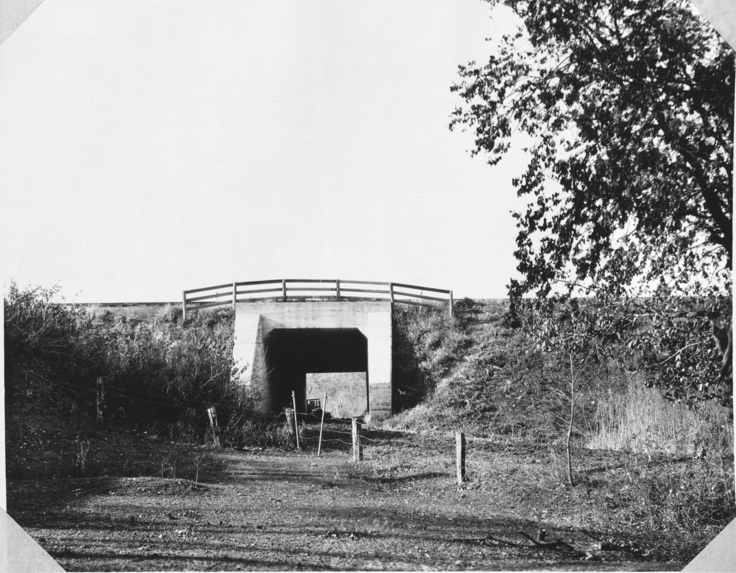
View No. 6 Line A Underpass in Ashland opposite Station 959, 250' from recommended route.
