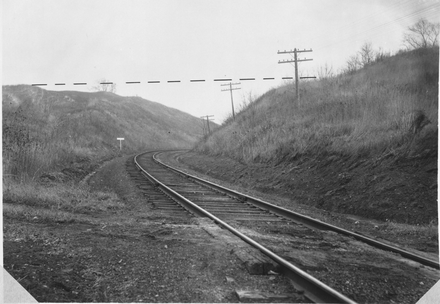
View No. 7 Line A Site of overhead crossing over Louisville line of Burlington Railroad, Sta. 1042.
