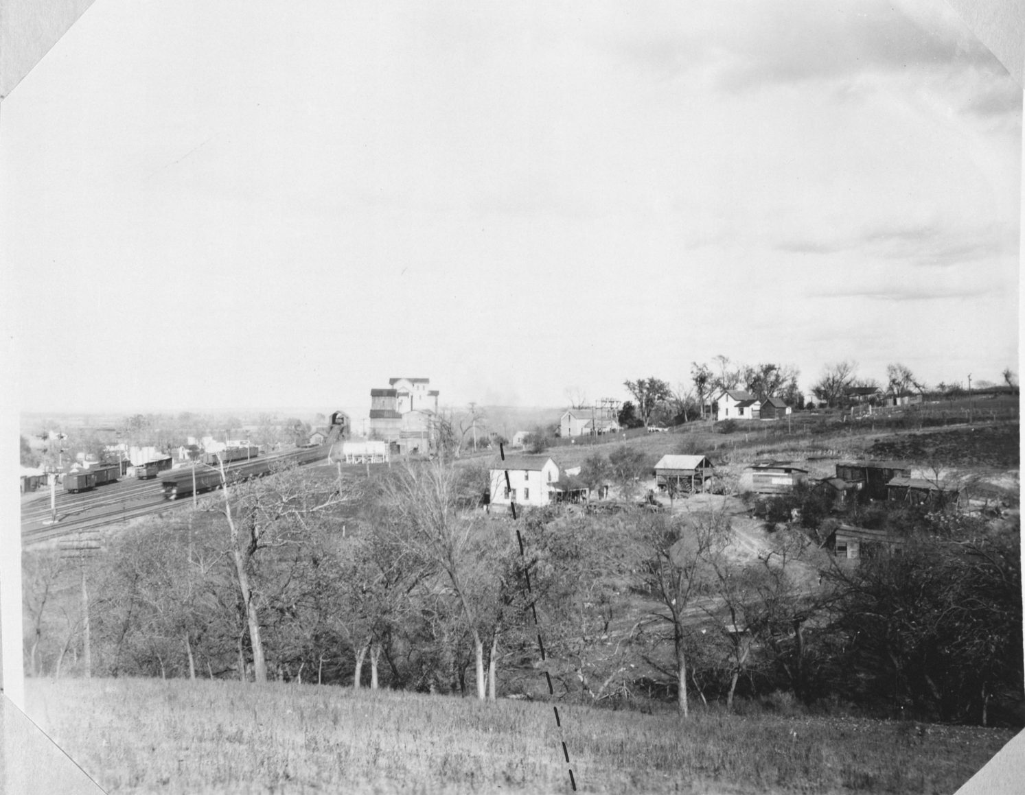
View No. 2 Line A Looking east through Ashland from Station 956.
