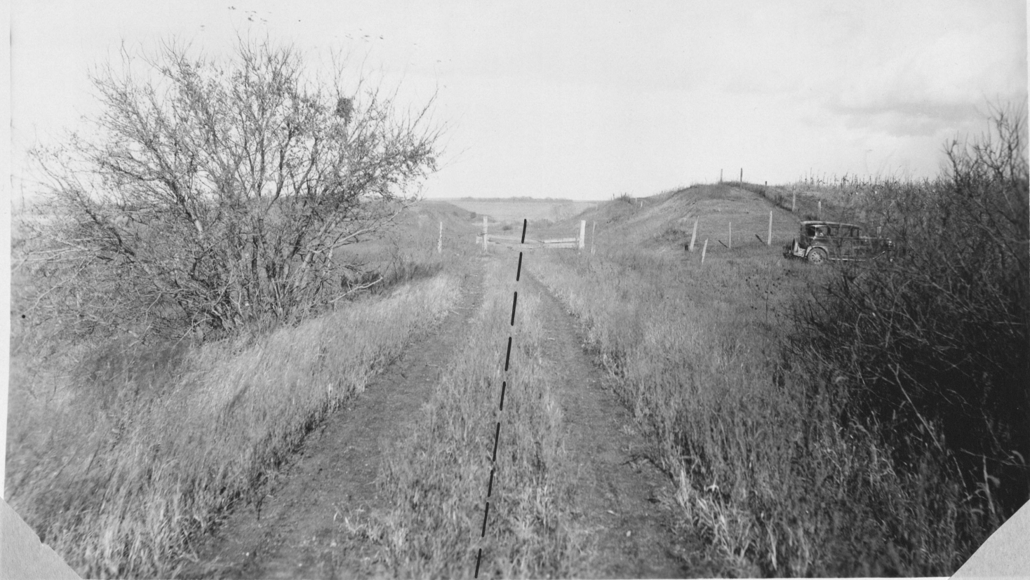
View No. 1 Line A Station 872 looking east on old railroad fills.
