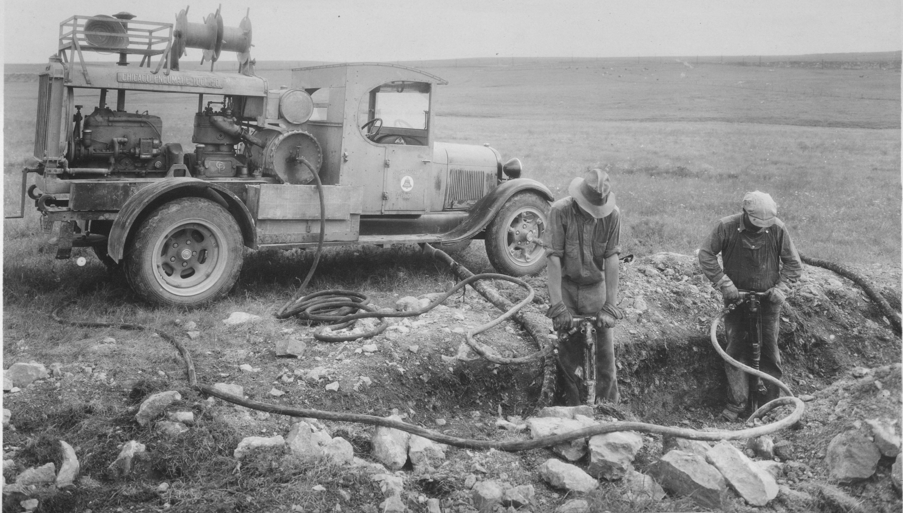
Figure 22. Compressed Air Drilling Apparatus.
