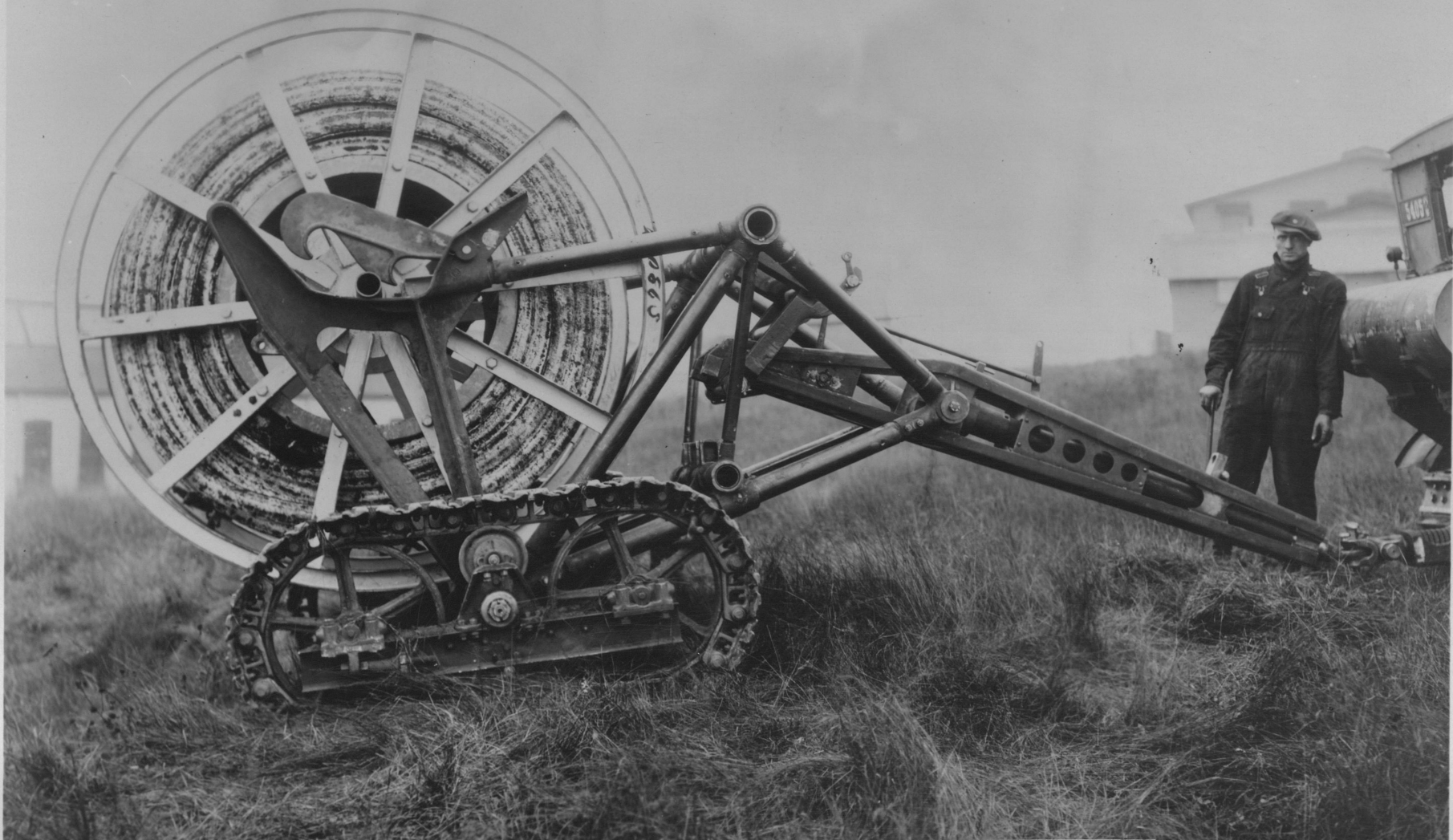
Figure 30. Traction Loading Cable Reel Trailer. Completion of Loading Operation.
