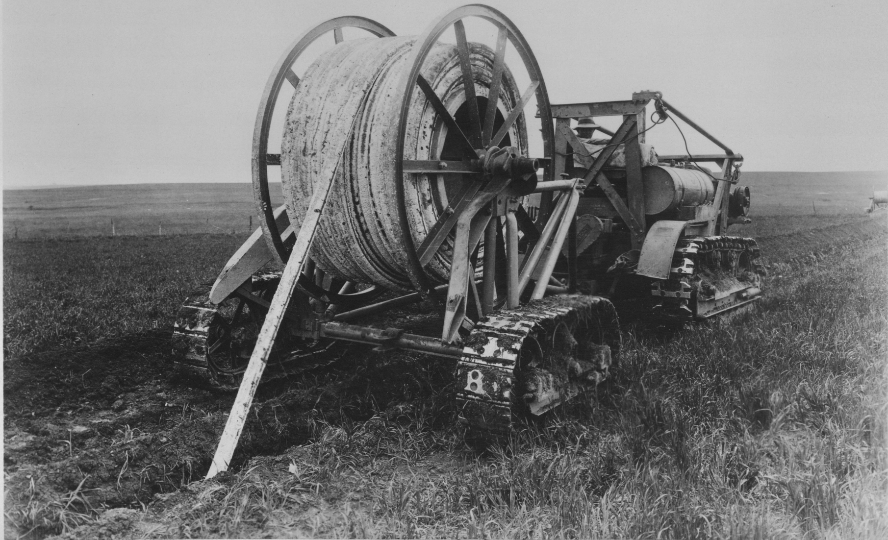
Figure 38. Laying Tape Armored Cable - One Trailer.
