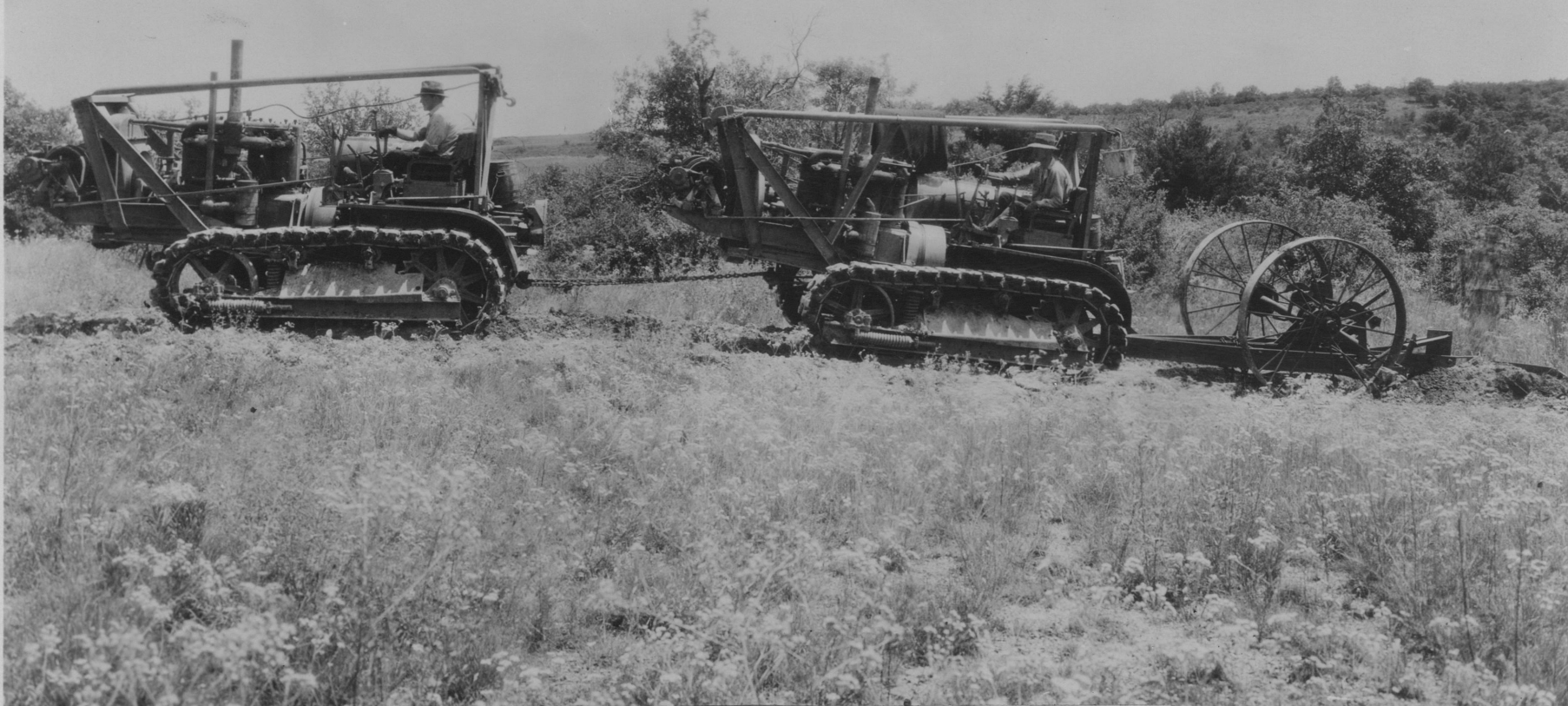
Figure 36. Trenching Plow in Operation.
