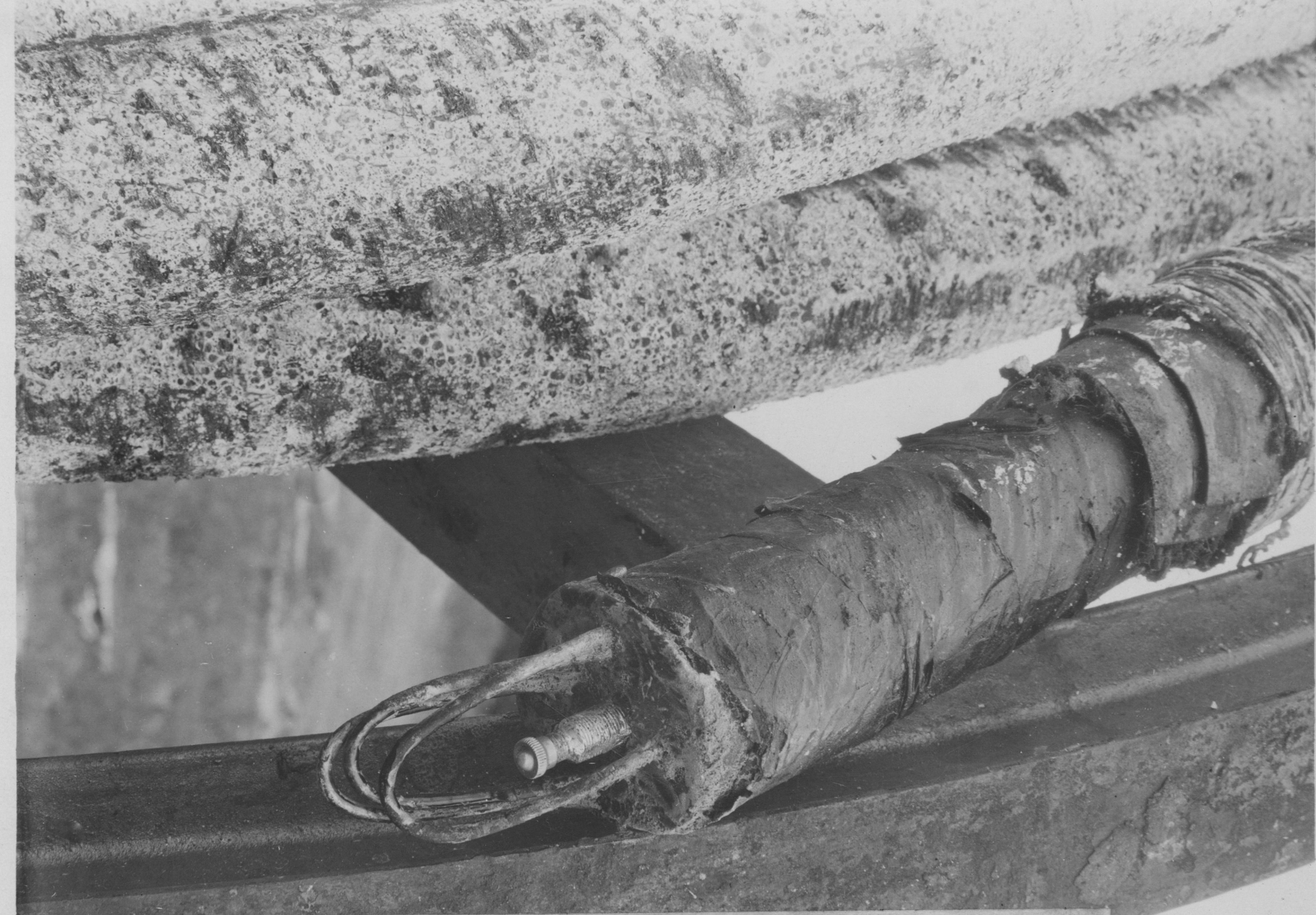
Figure 44. Gas Valve in End of Length of Tape Armored Cable.
