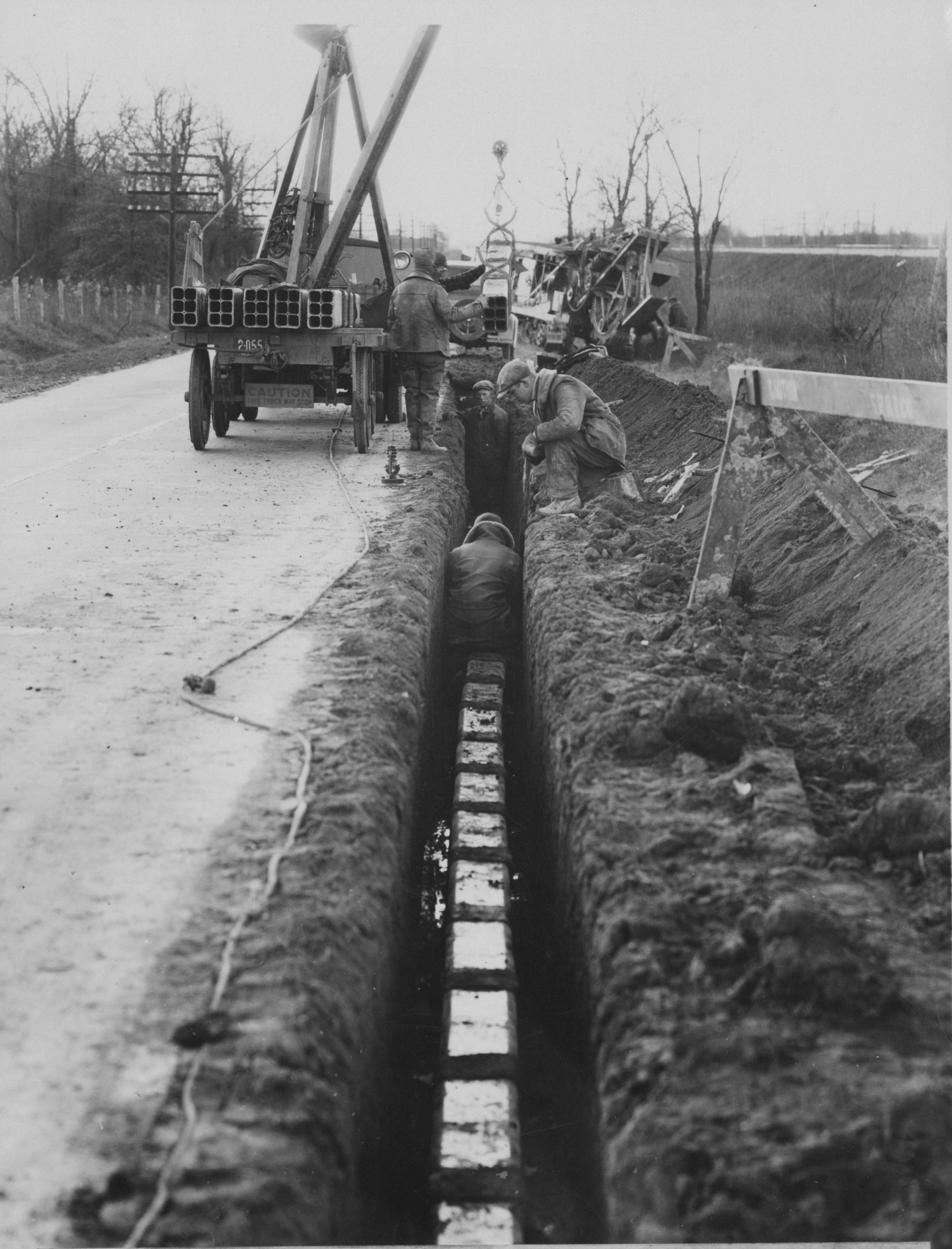
Figure 15. Installing 12-Foot Section of Conduit in Trench.
