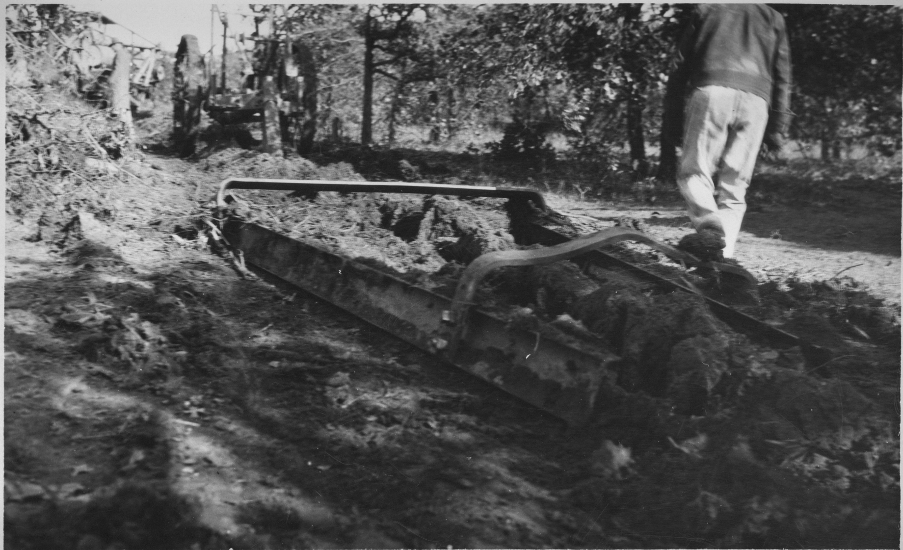
Figure 42. Backfiller - I-Beam Type.
