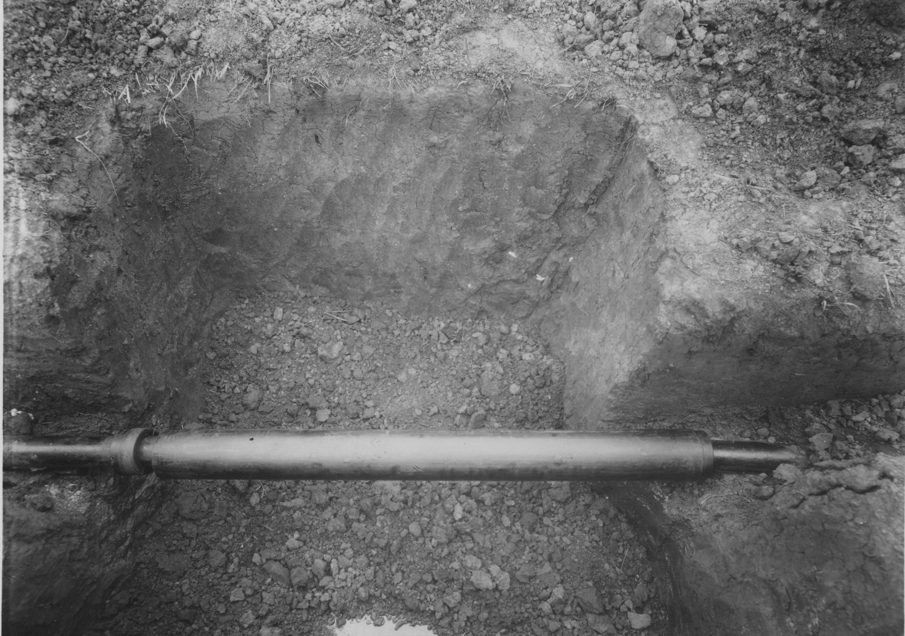
Figure 16. Fiber Splice Covering.
