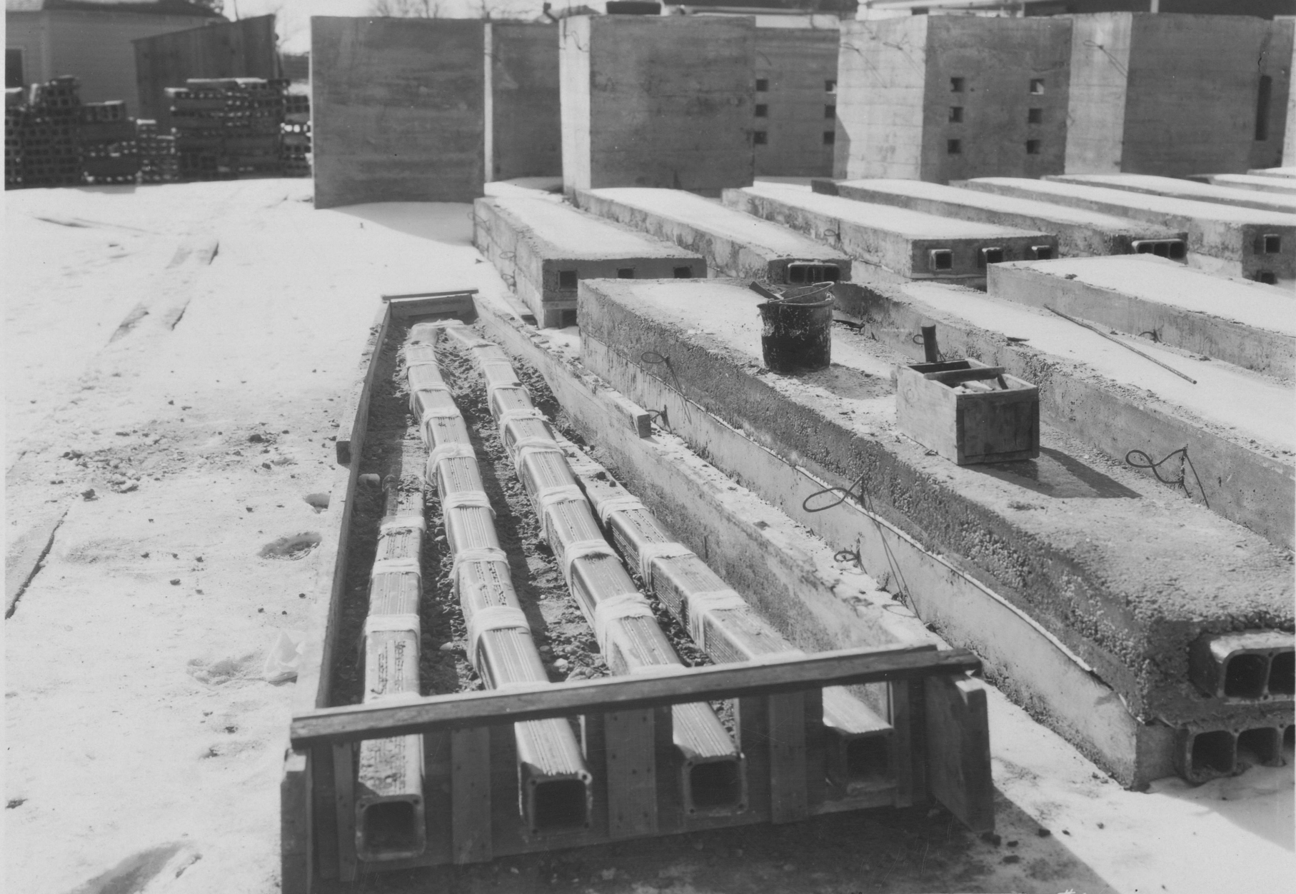
Figure 10. Form for Making Pre-Cast 4-Duct Splay.
