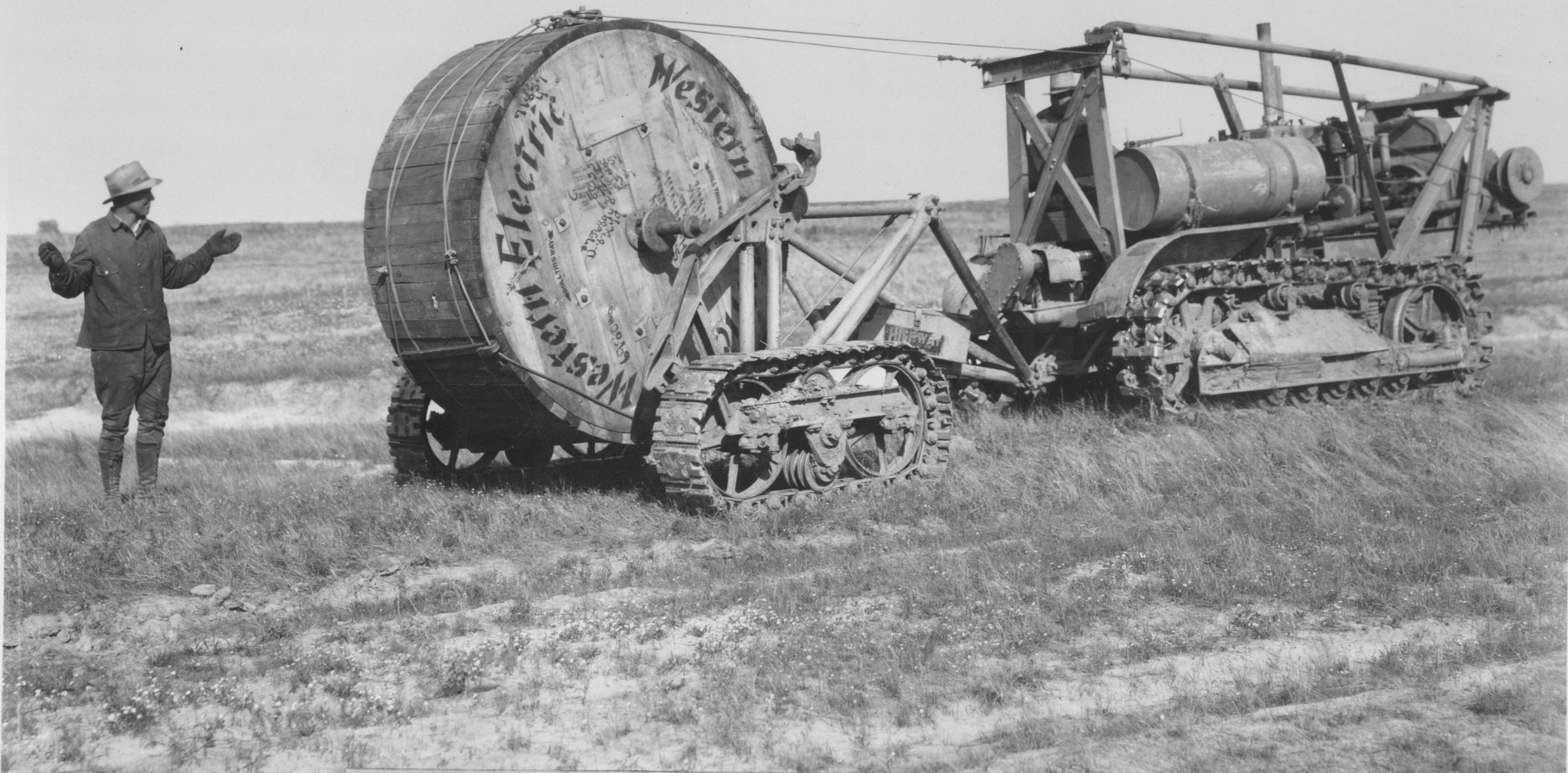
Figure 26. Loading Wooden Cable Reel on Trailer.
