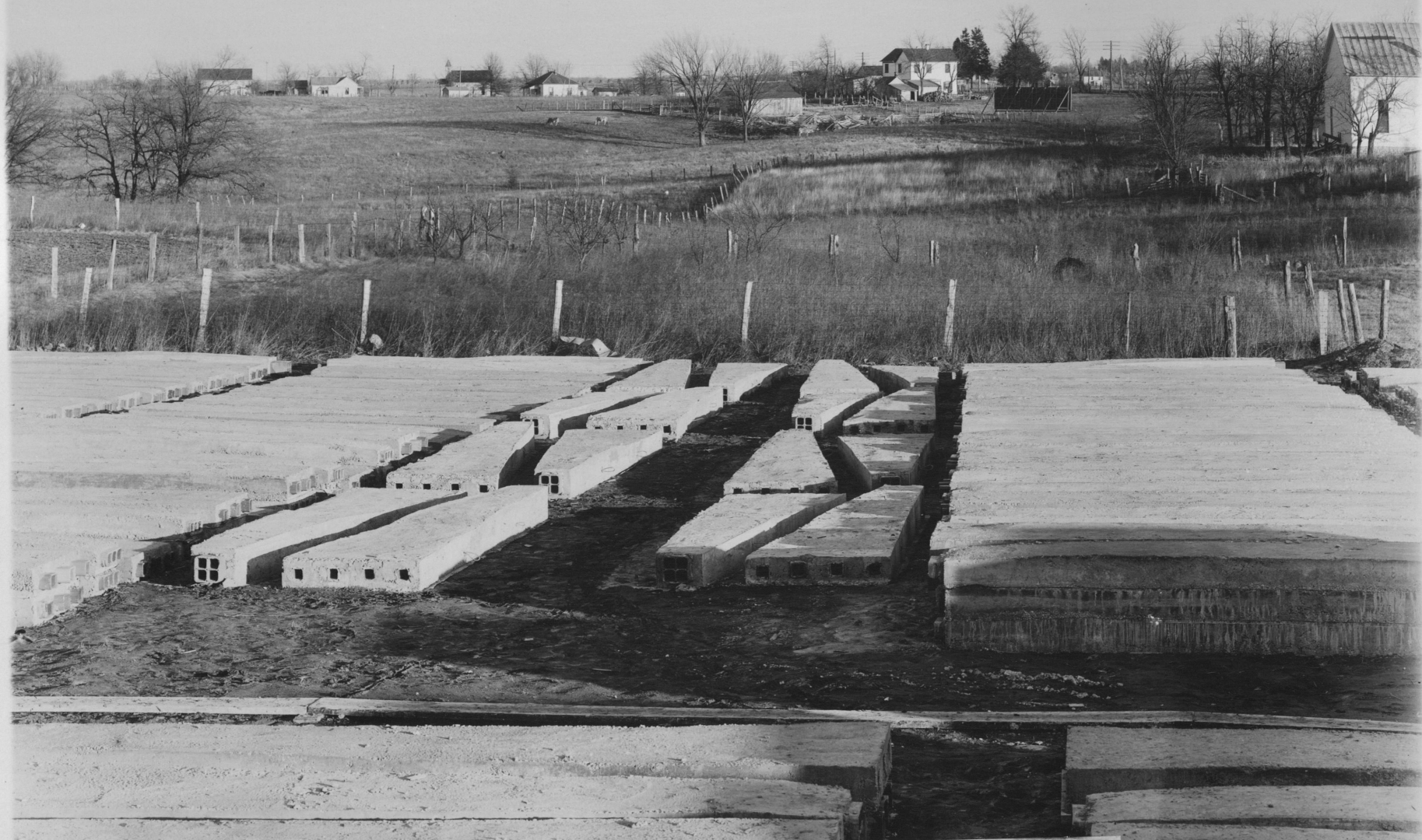
Figure 11. Completed Pre-Cast 4-Duct Splays.
