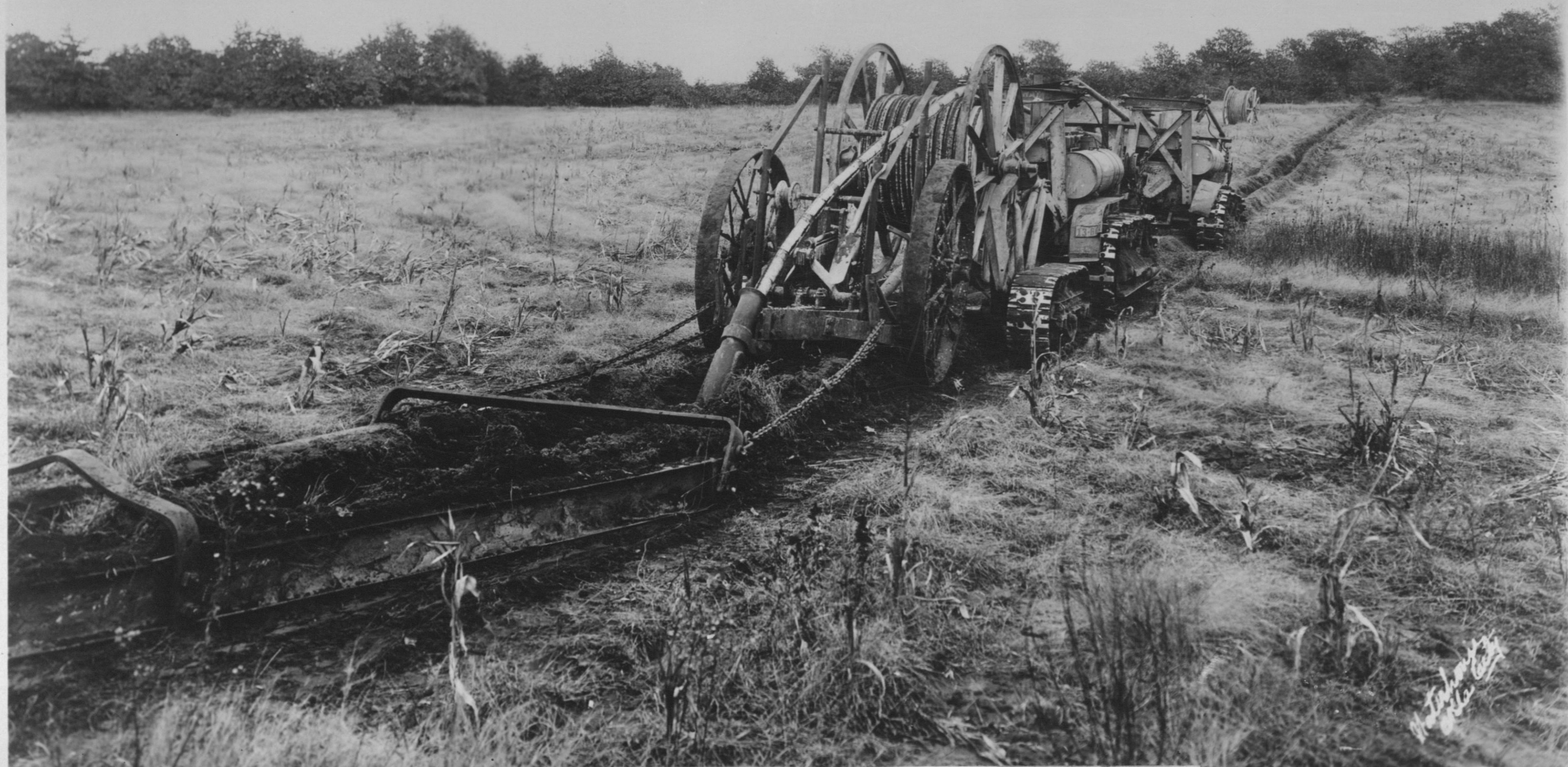
Figure 41. Cable Laying Plow in Operation.
