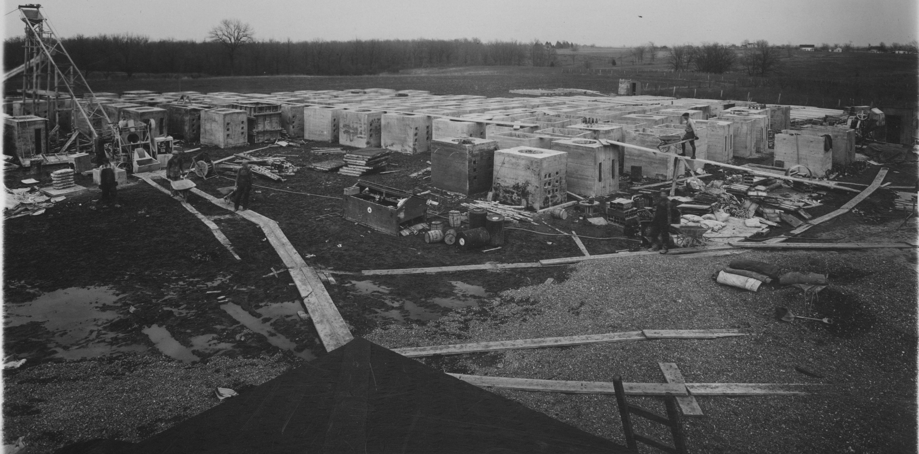
Figure 6. Manhole Pre-Casting Plant.
