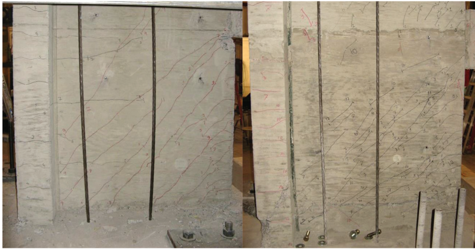
(a) Specimen CW-1 (reinforced concrete)
