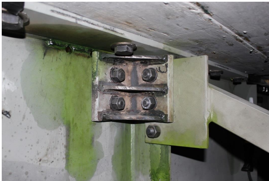
Figure 6: Stiffened angles-with-plate retrofit applied to exterior girders in Trials 1.7 and 2.2-2.7.
