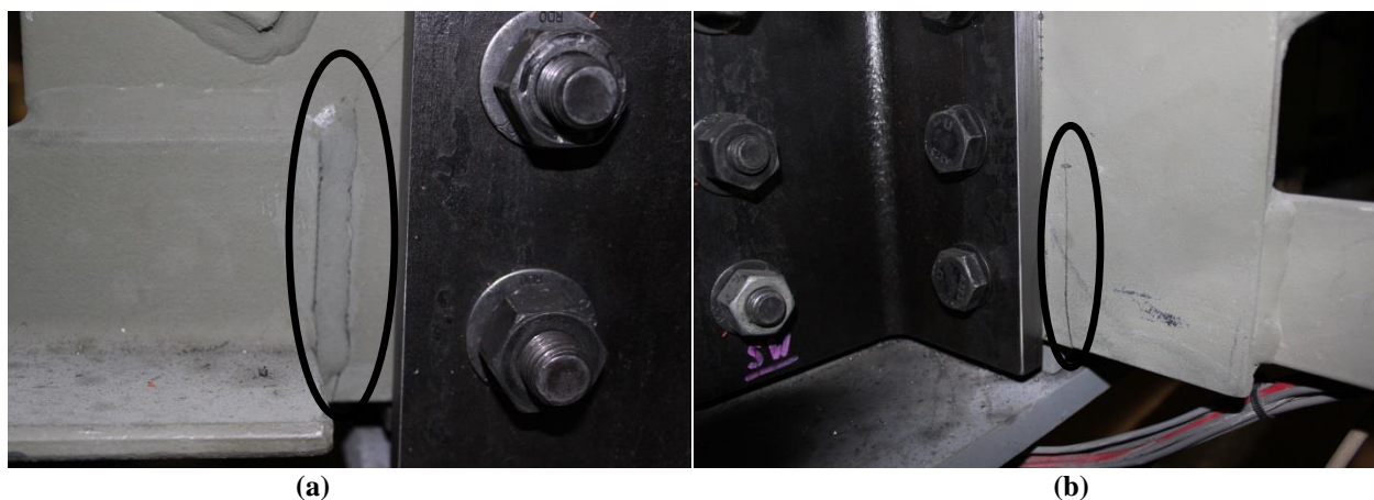
Figure 18: South cross frame tab plate failure from (a) east and (b) west side of cross frame.
