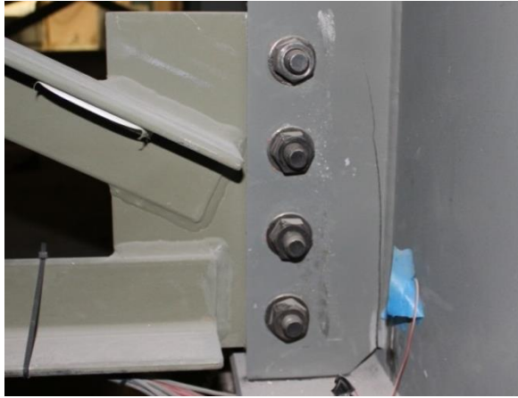
Figure 16: Crack found in cross frame connection plate at the south face of the center girder.
