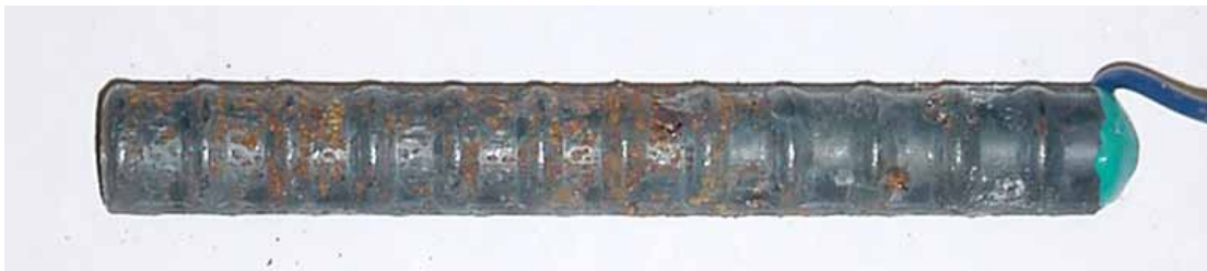
Figure 10. Photo. Bare conventional anode bar, at 15 weeks, showing corrosion products that formed below the surface of the solution.
