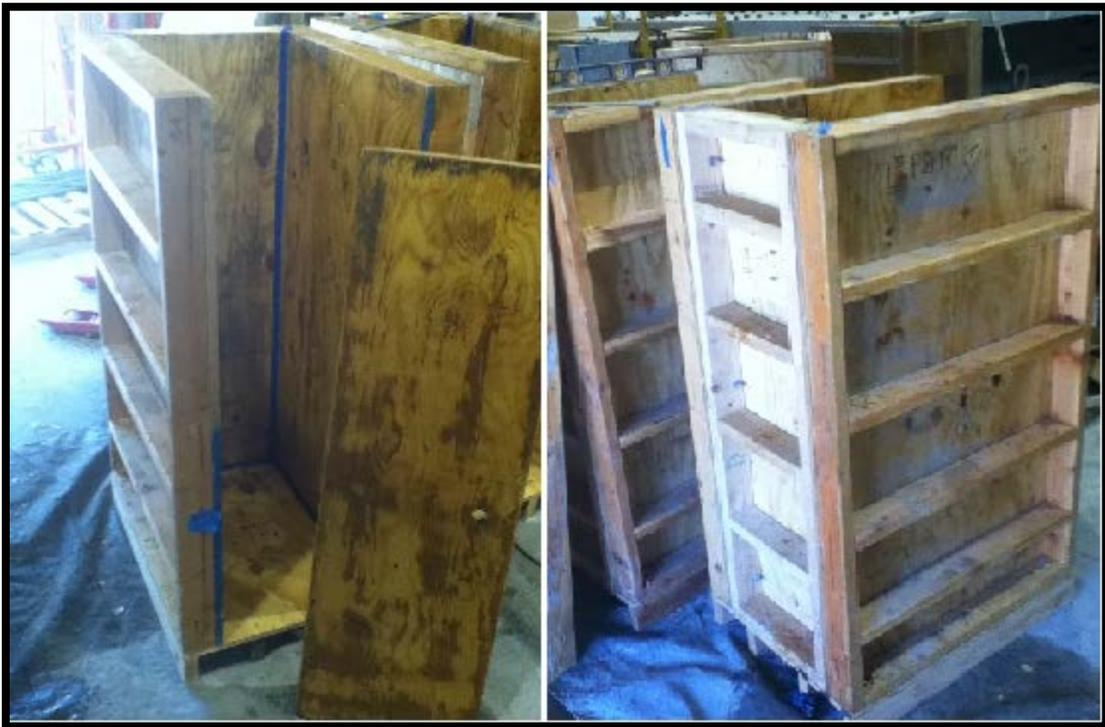
**Figure 6: Front and back view of forms**
