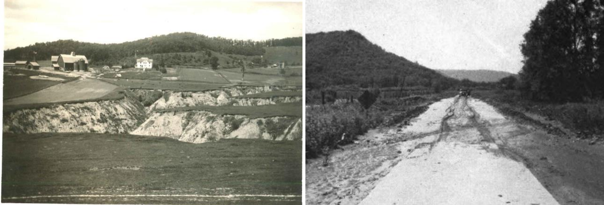
Figure 25: (Left) Gully on a farm owned by a man named McDonald in Alma, Wisconsin. Although Alma abuts the Mississippi River, it lacks any “bench terraces” and is thus more representative of the rest of the Driftless Area. (Right) Ten inches of sediment covering Minnesota State Highway No. 74 in Winona County, Minnesota, illustrating the types of highway sedimentation problems Otto Zeasman encountered in the 1920s. Sources: Otto R. Zeasman Papers, University of Wisconsin Archives (photo by Gottlieb Muehleisen); Stafford C. Happ, et al., Some Principles of Accelerated Stream and Valley Sedimentation , Technical Bulletin No. 695 (Washington, D.C.: USDA, May 1940), Plate 13B.
