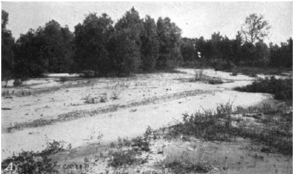
Figure 35: (Top) A drainage ditch in the Wells drainage district completely filled with sand, Lafayette County (ca. 1937). (Bottom) A sand splay in an abandoned field adjacent to the filled ditch pictured above. Source: Happ, et al., Some Principles of Accelerated Stream and Valley Sedimentation , Plates 5-A, 7-A.
