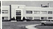
New plant construction has returned to the Muskingum Valley. Here, a new factory building for the nation's largest manufacturer has been planned on 100 acres of land. Thousands of new jobs have been created, restoring the economy of the Valley.
