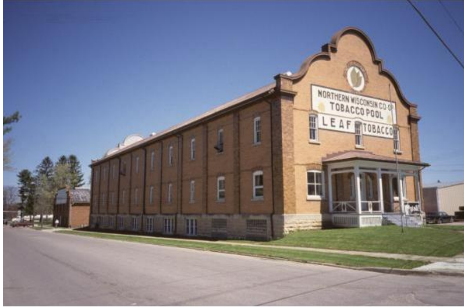
Figure 32: The Northern Wisconsin Co-Op Tobacco Pool building (constructed in 1906) in Viroqua, Wisconsin, stands as a legacy to the importance of tobacco farming in the Driftless Area—particularly in Vernon County, Wisconsin—during the twentieth century. Two buildings nearby (one of which is visible behind the featured building) were also used to cure, store, and market Driftless Area tobacco. Source: Wisconsin Historical Society.
