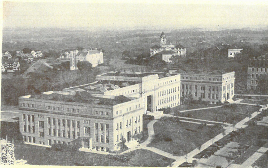
Administration Building As the View Appears from Atop the Radio Tower
