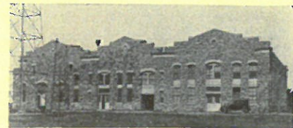
Added Electrical Lab in '22
