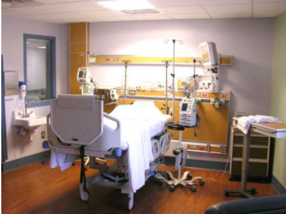
Figure 8: Headwall in a patient room.
