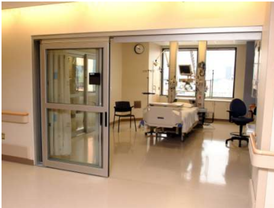
Figure 11: Patient room with a glass breakaway door.
