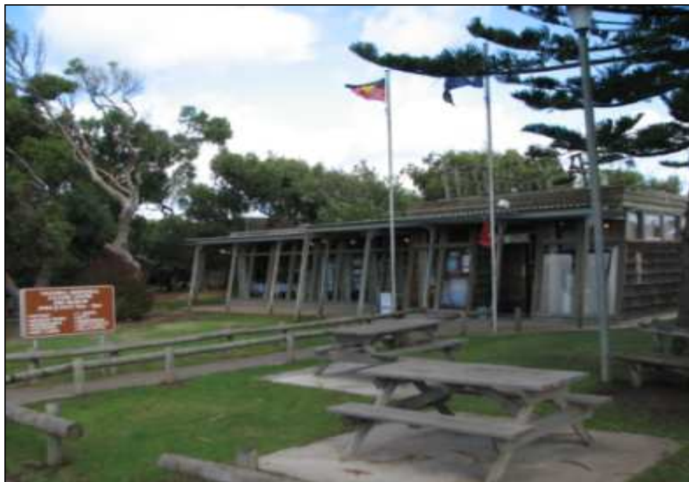
Figure 8.9: Exterior of the Tiagarra Aboriginal and Cultural Centre in Devenport (photo taken by author)
