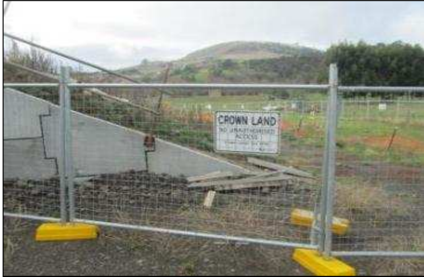
Figure 8.2: Fences erected at the Brighton Bypass Bridge site (photo taken by author)
