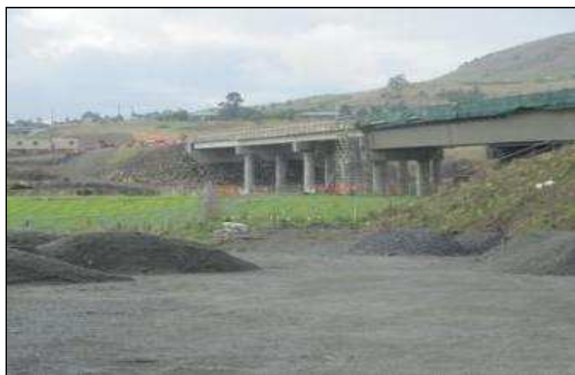
Figure 8.1: The Brighton Bypass Bridge under construction (photo taken by author)
