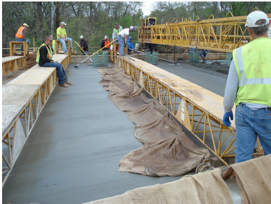
Figure 5.25 Burlap drag used for finishing on OP Bridge Placement 2
