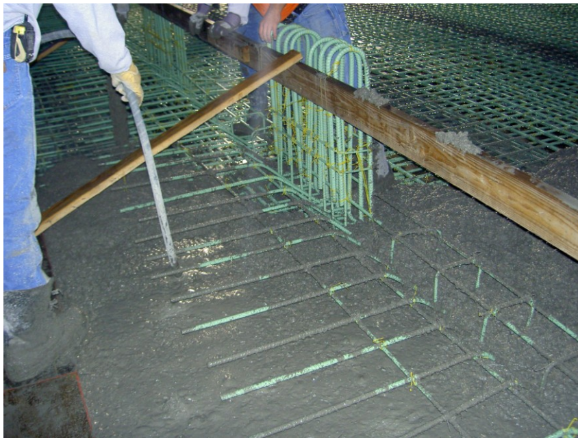
Figure 5.5 Hand-vibration near reinforcement bars – LC-HPC-2
