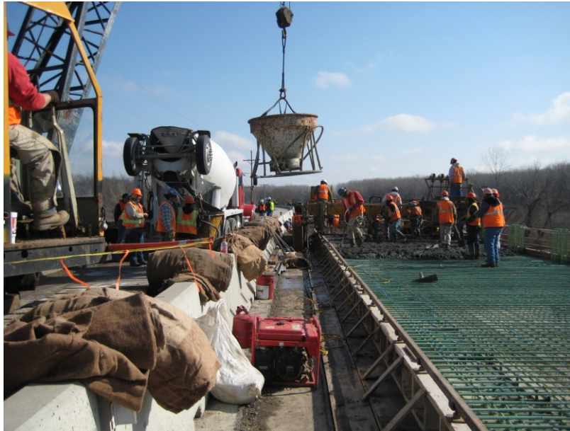
Figure 5.18 Equipment orientation and placement method for LC-HPC-12 Placement 1
