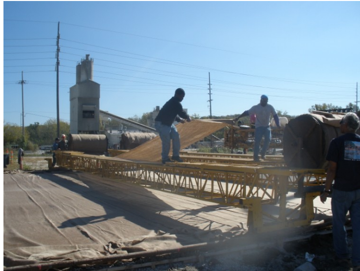
Figure 5.26 Pre-cut, pre-rolled burlap placed on qualification slab for LC-HPC-16
