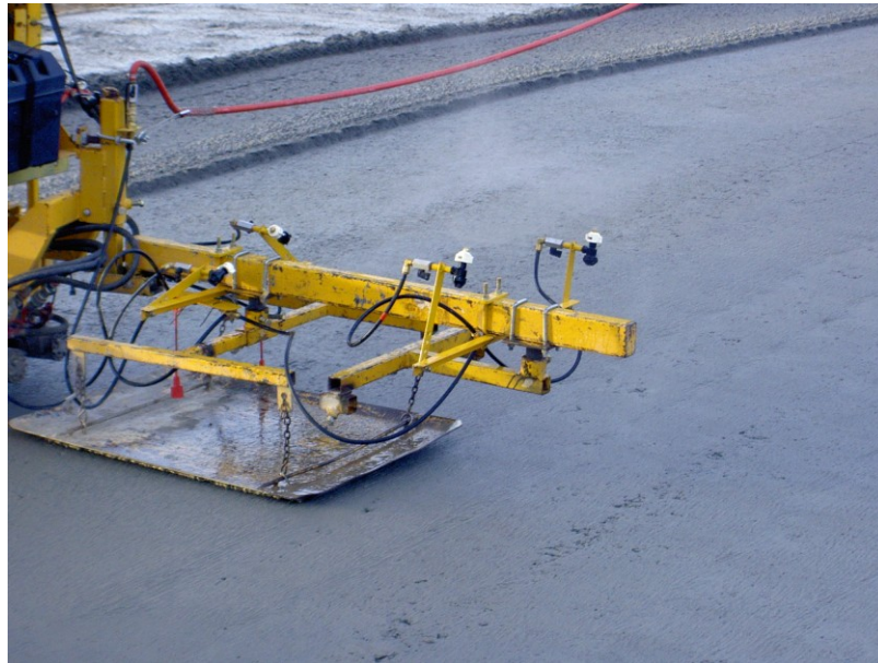
Figure 5.7 Fogging system placed on pan drag – LC-HPC-7 qualification slab
