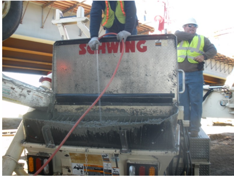
Figure 5.27 Water added to hopper to aid pumping – LC-HPC-16
