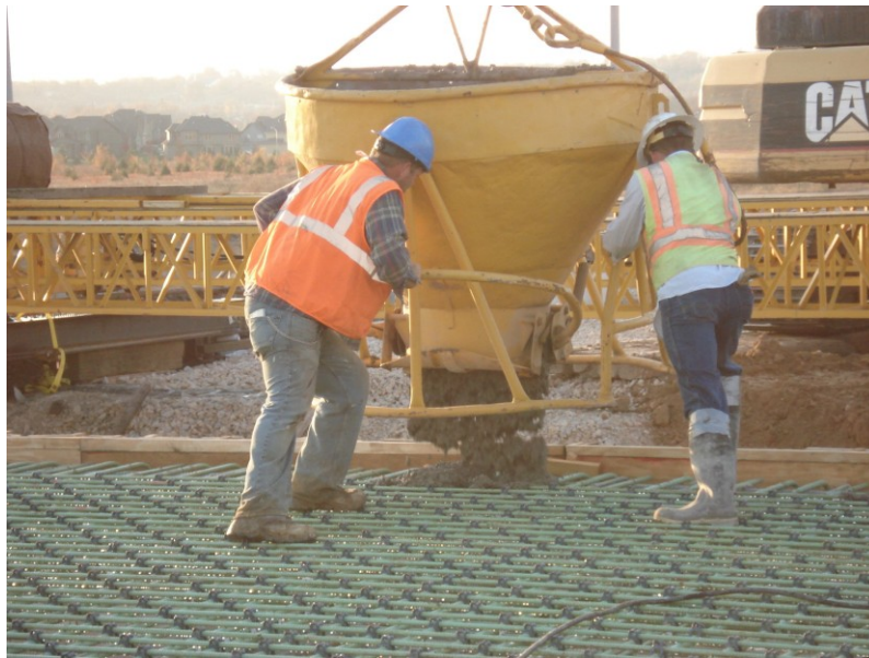
Figure 5.29 Concrete placed by crane bucket for LC-HPC-15
