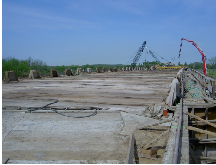
Figure 5.10 Dry burlap covering deck – LC-HPC-10
