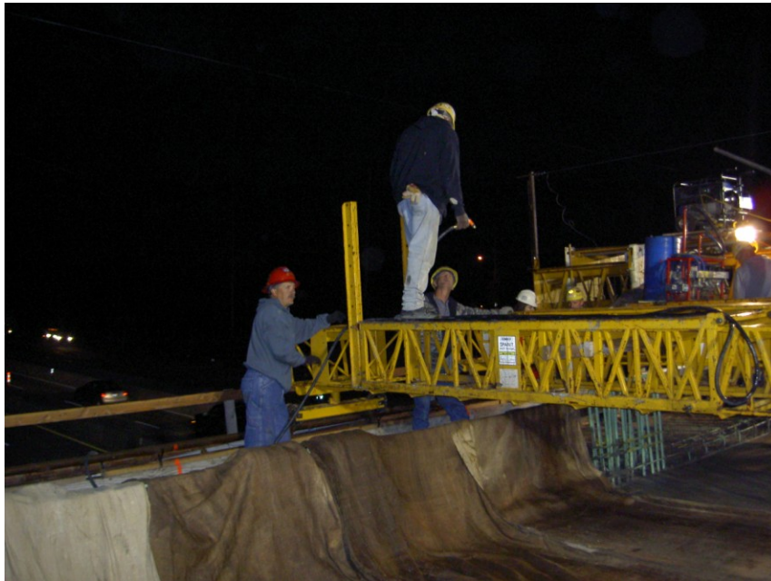
Figure 5.6 Contractor used sprayed water as a finishing aide – LC-HPC-2
