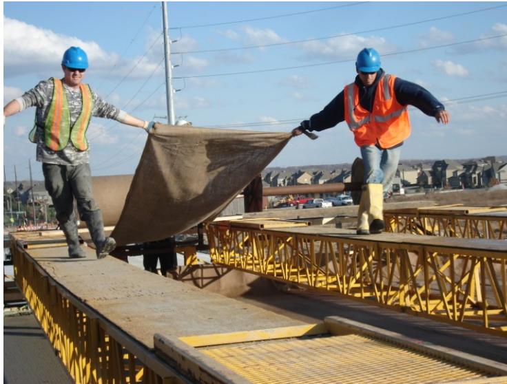
Figure 5.30 Burlap placement on LC-HPC-15
