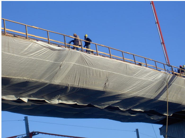
Figure 5.16 Girders wrapped for requirements of cold-weather curing – LC-HPC-6
