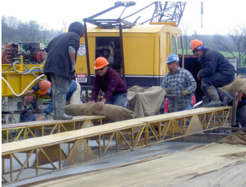
Figure 5.9 Contractors experienced difficulties placing folded burlap – LC-HPC-10 qualification slab
