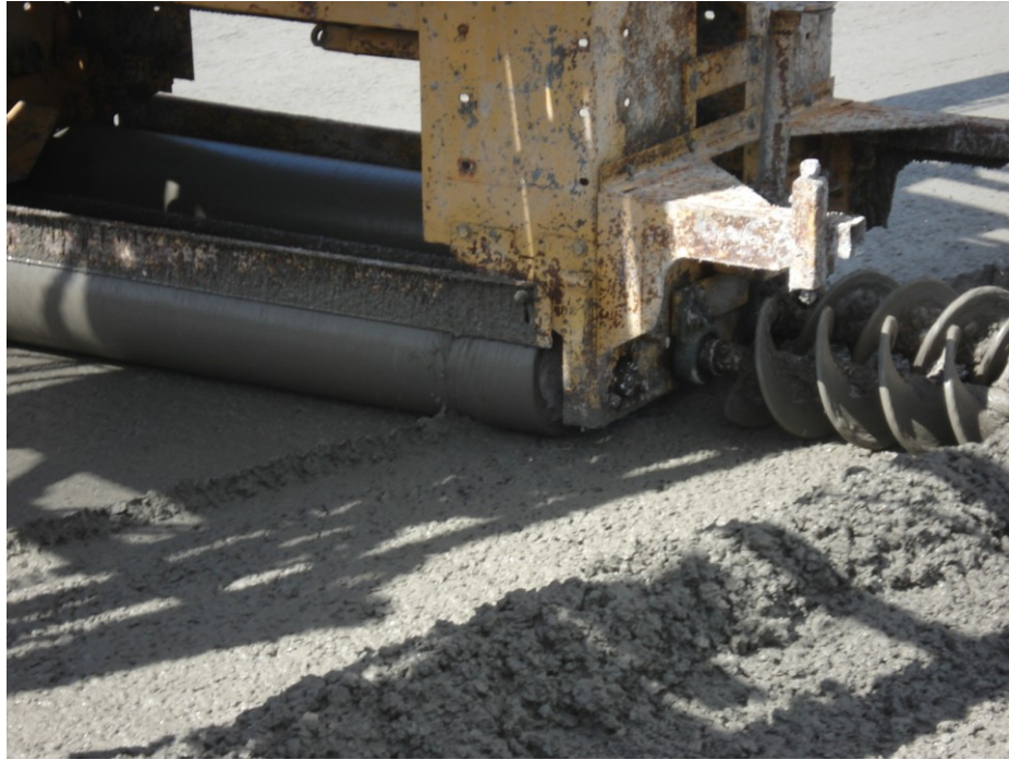
Figure 5.24 Double drum-roller screed used for finishing on OP Bridge Placement 2
