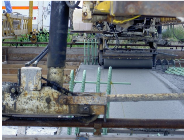
Figure 5.1 Single-drum roller screed – LC-HPC-1 qualification slab
