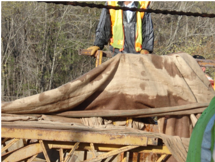
Figure 5.21 Partially-dry burlap – LC-HPC-9
