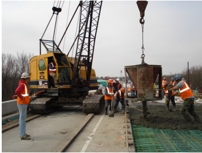
Figure 5.19 Construction equipment placed on newly-constructed Placement 1 during construction of LC-HPC-12 Placement 2
