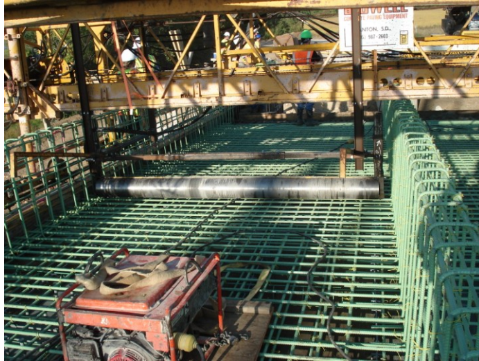
Figure 5.33 Single-drum roller screed used for strikeoff of sidewalks – LC-HPC-17
