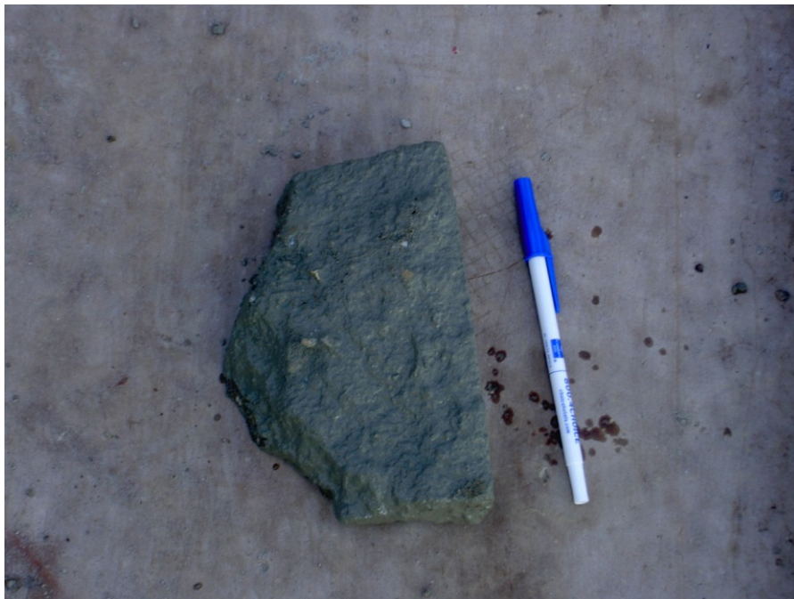
Figure 5.14 Large pieces of aggregate found in concrete during placement of LC-HPC-11
