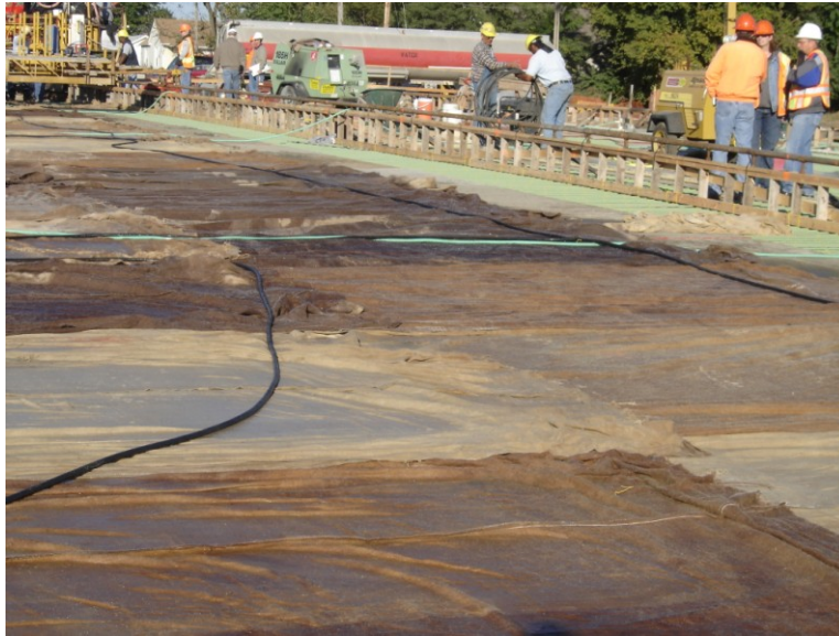
Figure 5.2 Soaker hoses placed on burlap – LC-HPC-1 Placement 1
