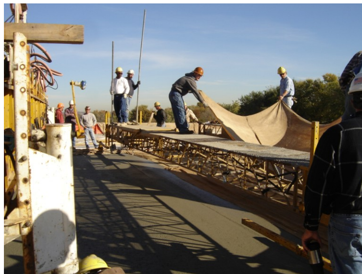
Figure 5.3 Burlap placement – LC-HPC-1 Placement 2
