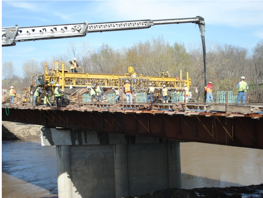
Figure 5.20 Height of concrete drop from second conveyor belt to deck – LC-HPC-9
