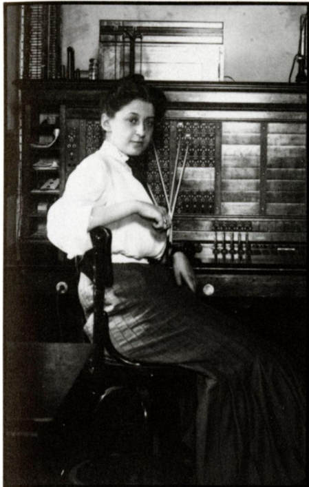
Fort Riley telephone exchange, 1905
