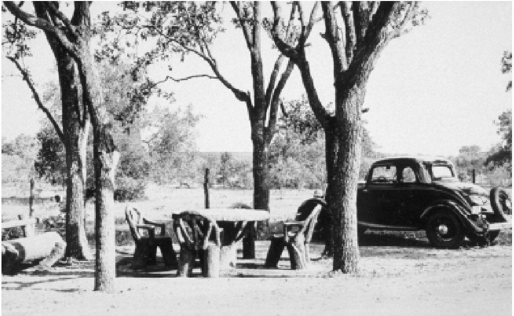
16. Tables and benches constructed from concrete to imitate natural logs, an art of reproduction known at that time only to a few Mexican Americans around San Antonio, roadside park, Wilson County, Texas, October 1934 (photo: courtesy of the Texas Department of Transportation)
