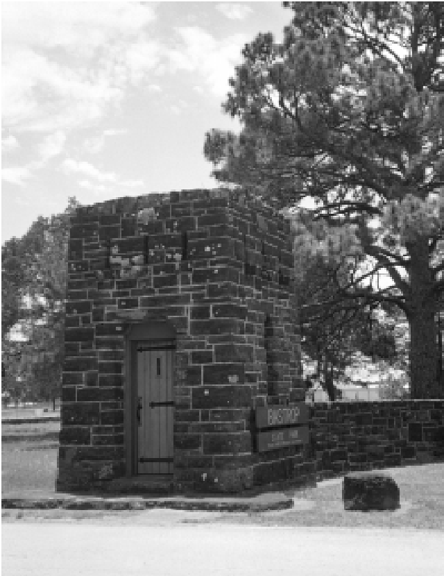
19. Park entrance gate at Bastrop State Park, Bastrop County, Texas, 1996
