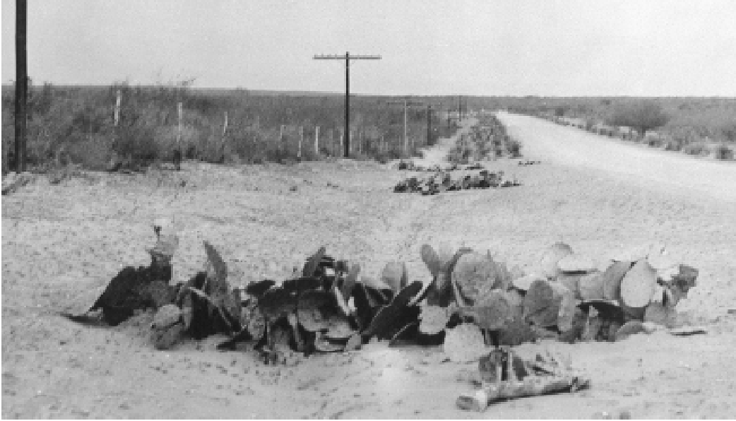
9. Native prickly pear cactus planted to retard ditch runoff, south Texas, December 1936 (photo: courtesy of the Texas Department of Transportation)
