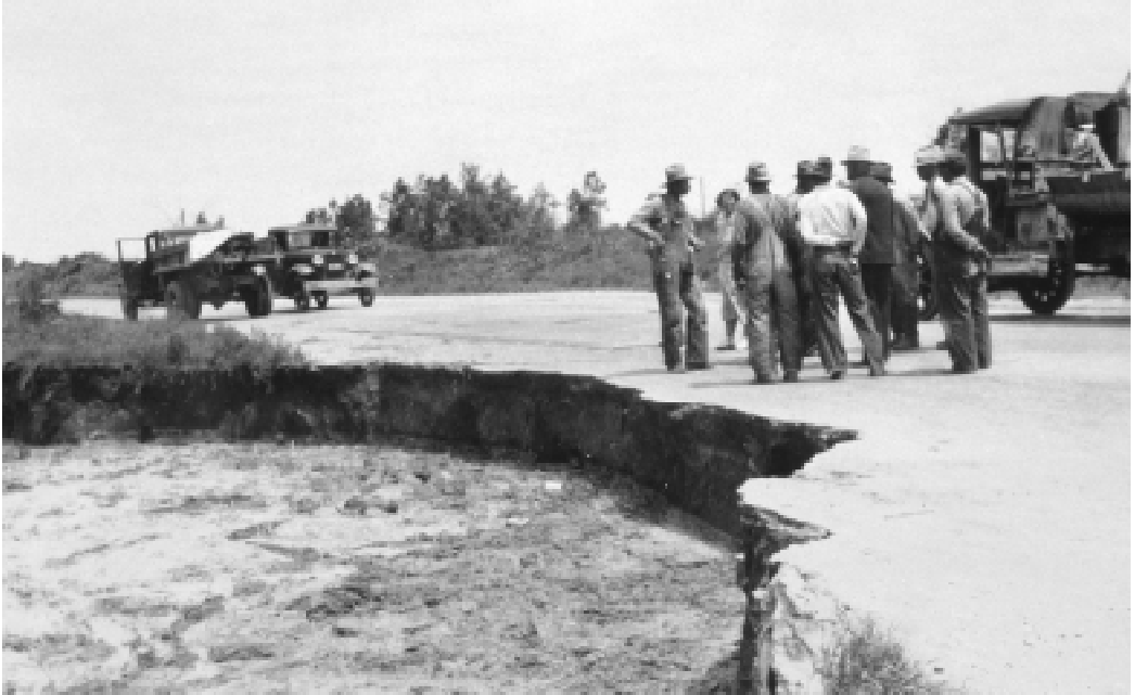
2. “What to Do?” Locals inspecting flood damage to a paved road in Dallas County, Texas, ca. 1936 (photo: courtesy of the Texas Department of Transportation)
