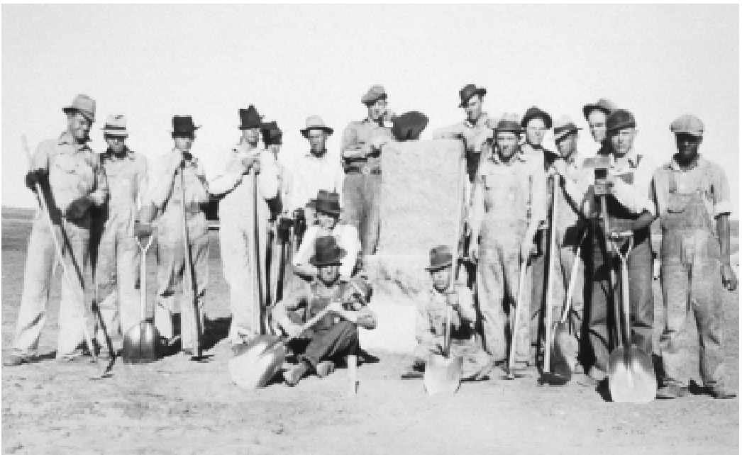
3. National Youth Administration work crew at Chisholm Trail Roadside Park, Wilbarger County, Texas, ca. 1937 (photo: courtesy of the Texas Department of Transportation)
