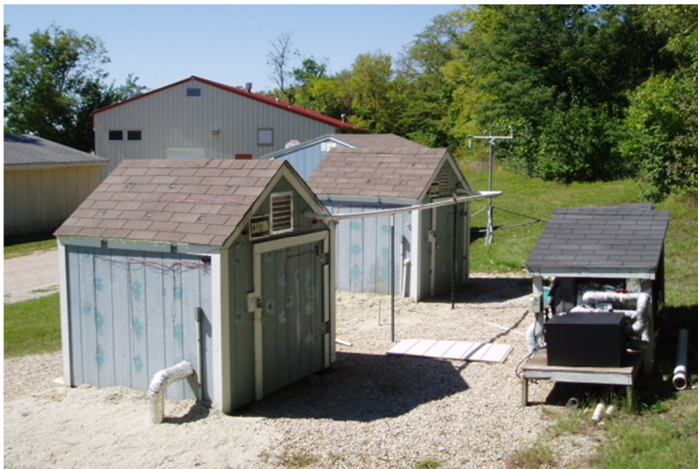
Figure 3.2. Test Houses - Back (North) and East Views
