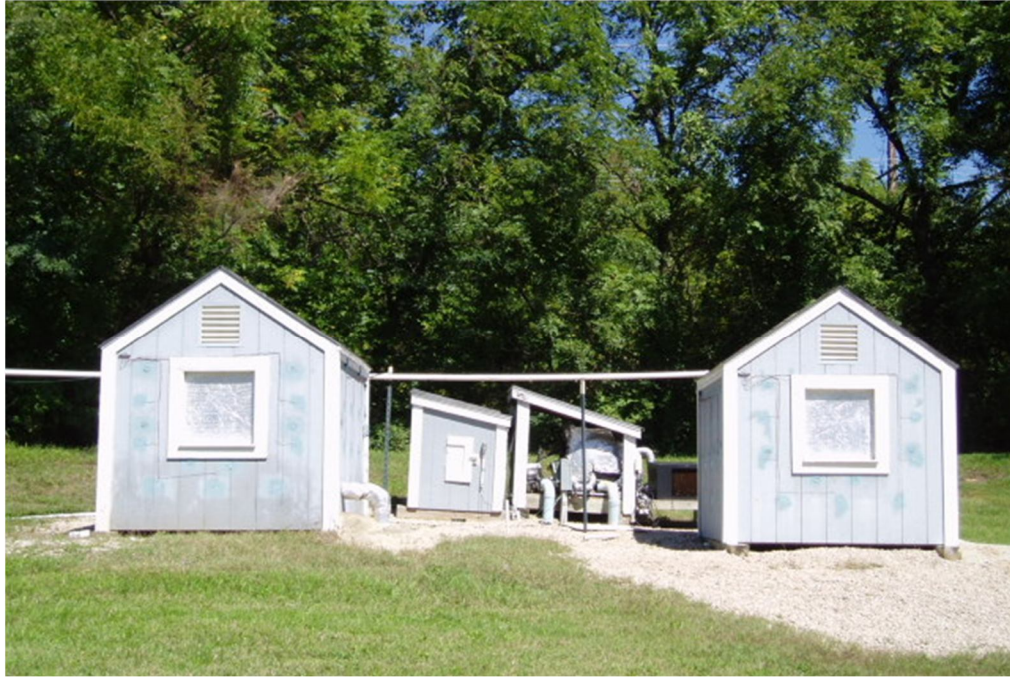
Figure 3.1. Test Houses - Front (South) View
