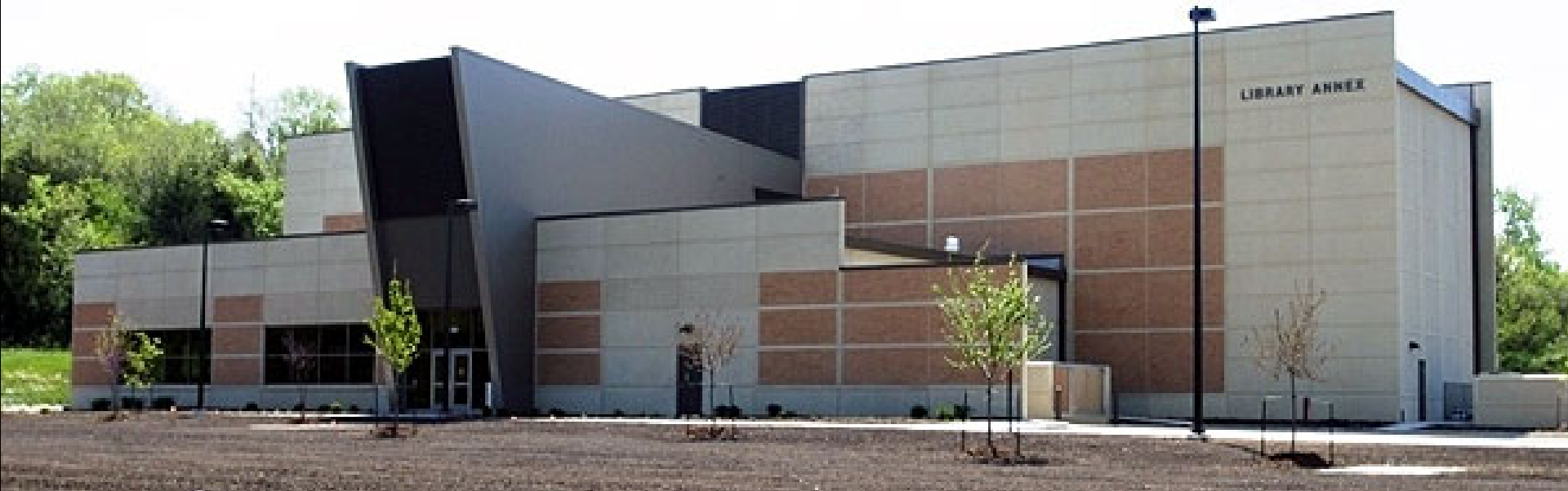
KU Library Annex
