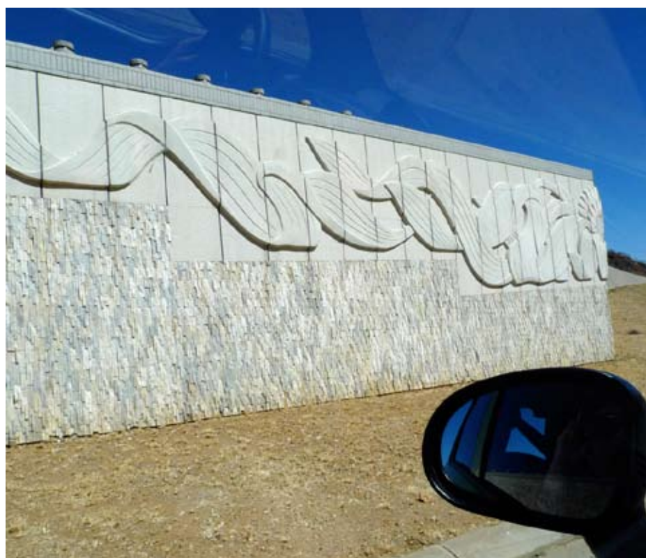
Figure 77: View of exterior wall and Welwitschia adornments, State House, Windhoek, Namibia.
