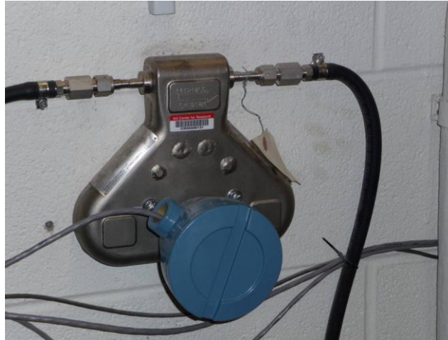
Figure 14. Fuel flow meter: MicroMotion CMF-010 coriolis flow meter.
