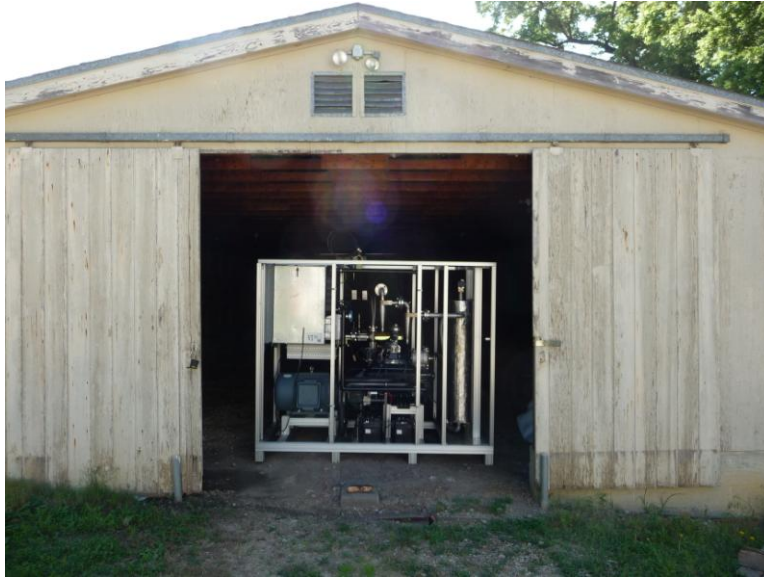
Figure 3. Temporary placement of the SynGas Rig in the boat barn.
