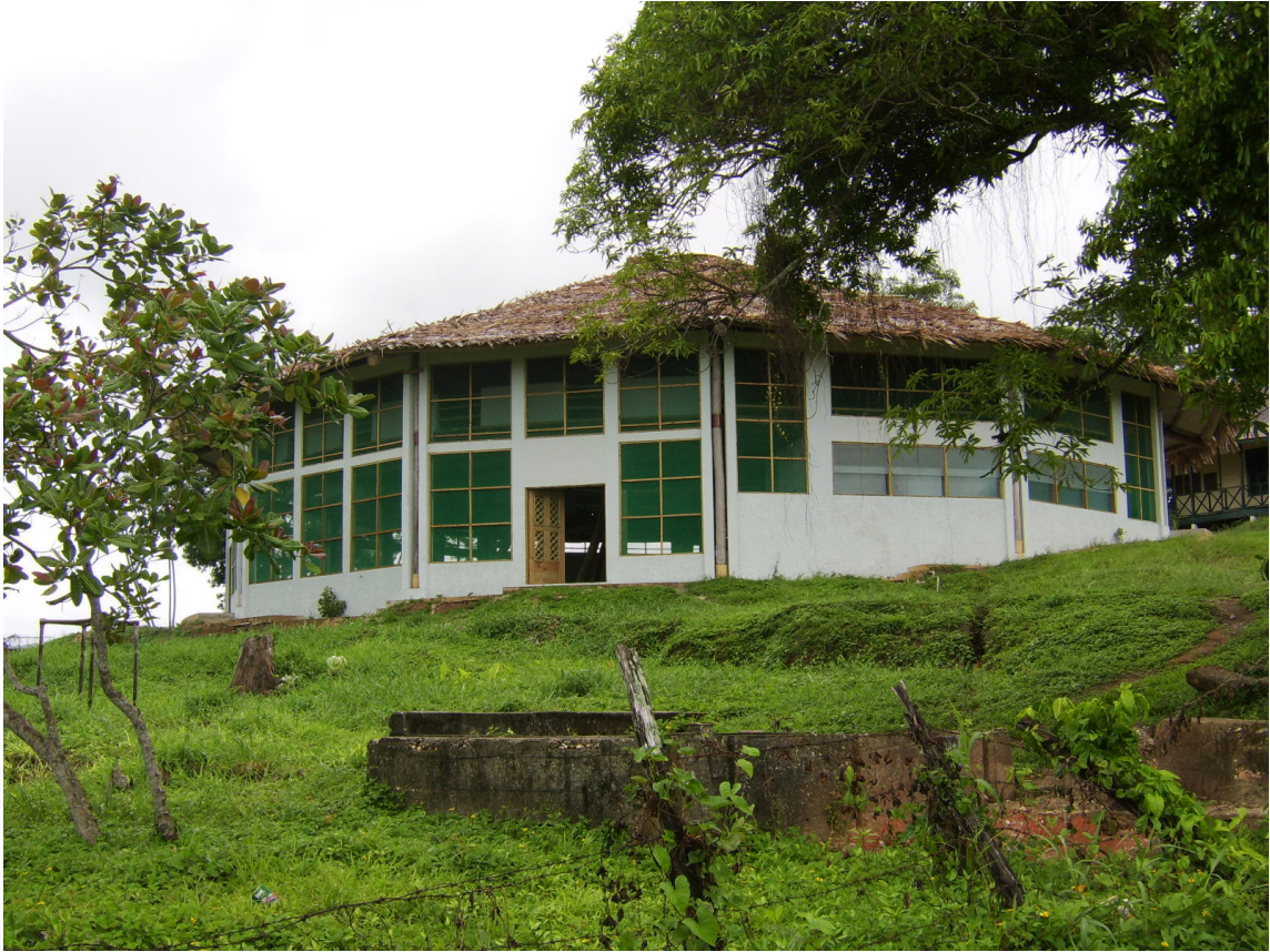
Garifuna Cultural Institute building (my photo, 2007).
