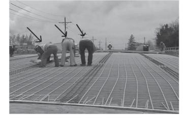
Fig. 2. An image of construction workers tying rebar for the concrete deck (image by Seonghoon Kim)
