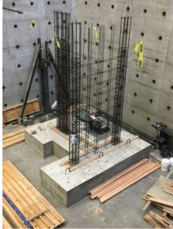
(b) Lift 1 steel cage
