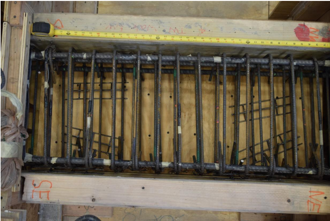
Figure B.4 – Coupling beam reinforcement, P100-2.5
