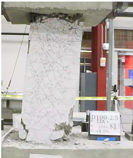
Figure C.48 – D100-2.5 at +8% chord rotation, first cycle
