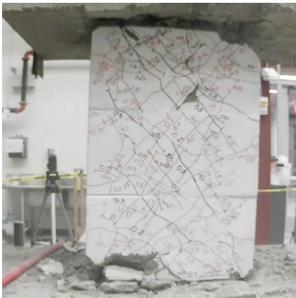
Figure C.19 – D100-1.5 at +8% chord rotation, first cycle
