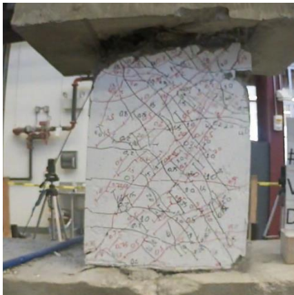
Figure C.24 – D120-1.5 at +4% chord rotation, second cycle
