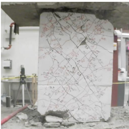
Figure C.15 – D100-1.5 at +8% chord rotation, first cycle
