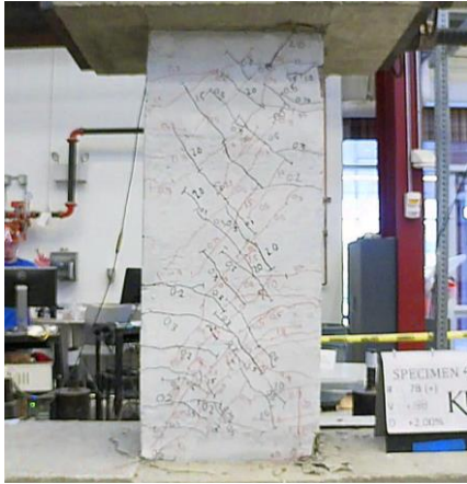
Figure C.22 – D80-2.5 at +2% chord rotation, second cycle
