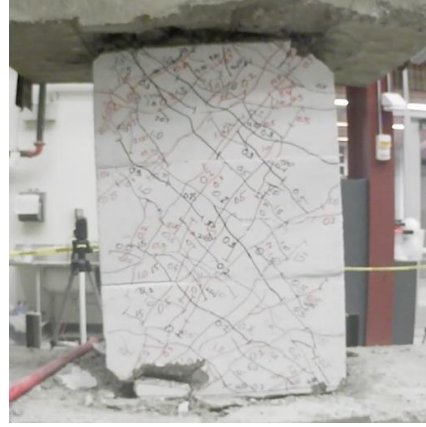
Figure C.14 – D100-1.5 at -6% chord rotation, second cycle
