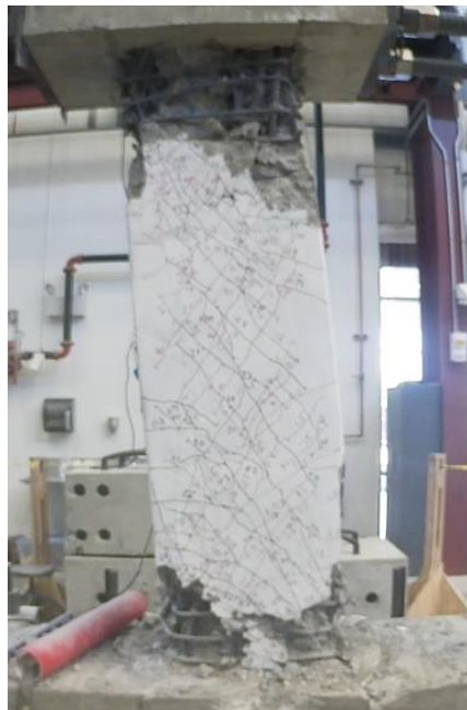
Figure C.55 – D80-3.5 at -8% chord rotation, second cycle
