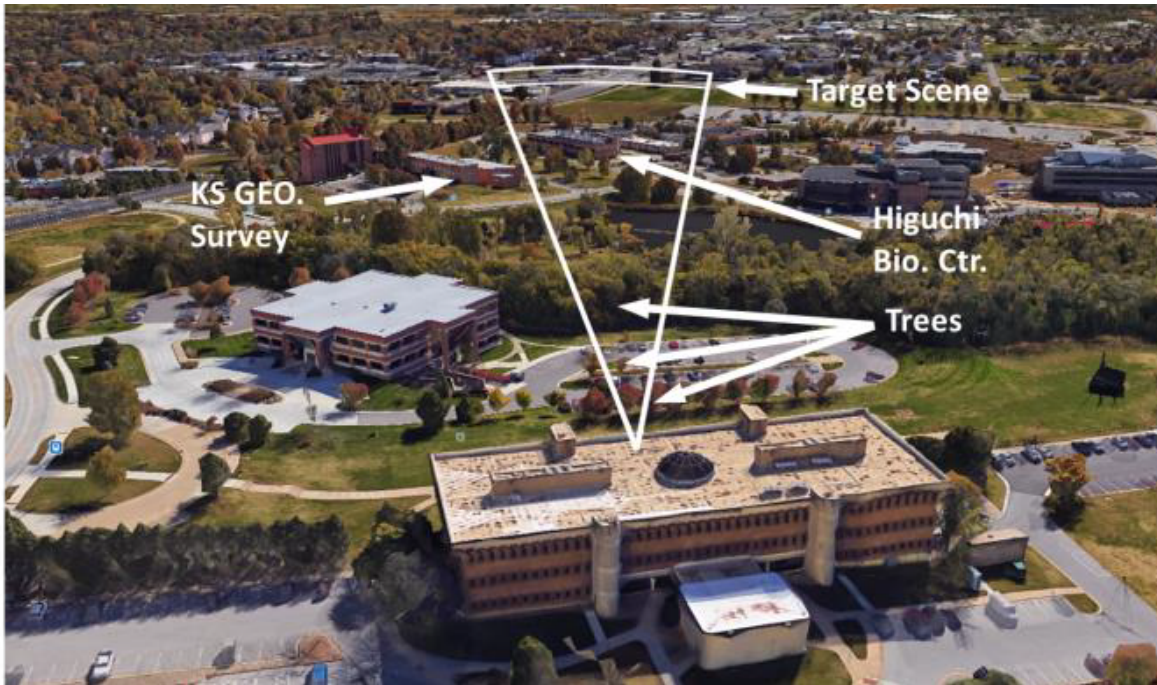
Figure 3.17: Aerial view generated using Google Earth depicting the roof of Nichols Hall and looking towards the 23rd and Iowa intersection.
